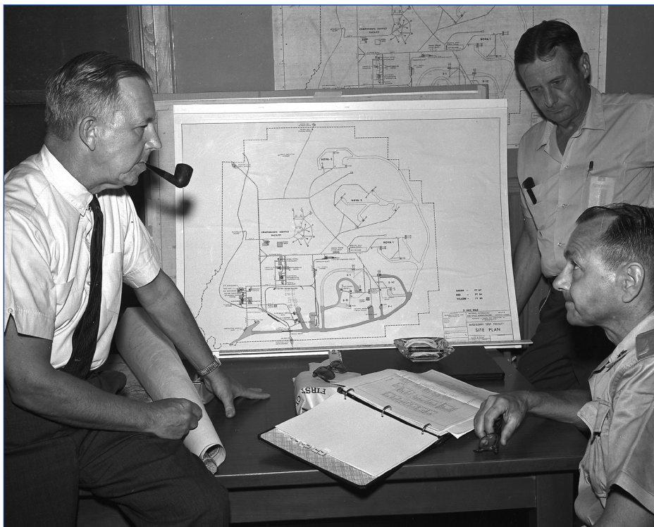
Capt. William C. Fortune (left), the first manager of Stennis Space Center, then known as Mississippi Test Operations, speaks with U.S. Corps of Engineers representatives Maj. Gen. Thomas Hayes (seated) and Charles Jackson during the early days of construction at the engine test site.
