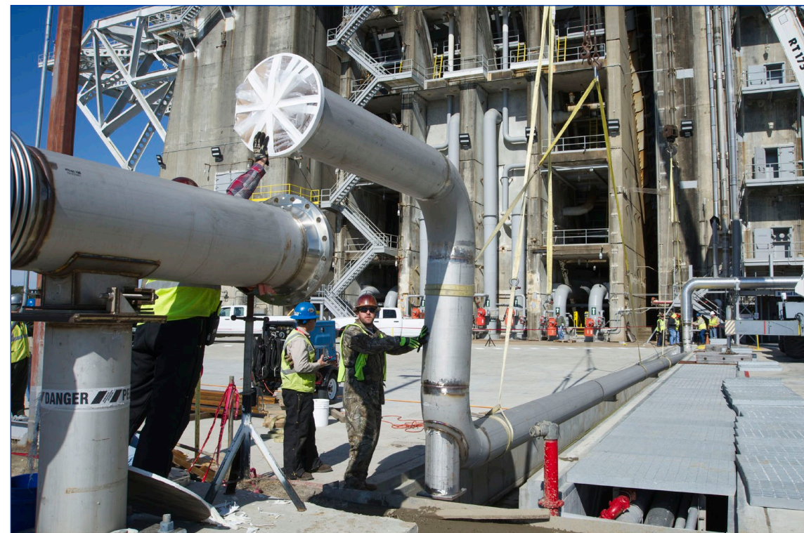
A work crew completes installation of an 18-inch-diameter hydrogen vent line at the B-2 Test Stand at Stennis Space Center early in February. Installation of the vent line, fabricated on site and installed by Syncom Space Services personnel, is part of preparations for testing the flight core stage of NASA's new Space Launch System rocket on the Stennis stand. Testing will involve installing the actual flight stage on the stand and firing all four of its RS-25 engines simultaneously, as during a launch. RS-25 engines burn a mixture of liquid hydrogen and liquid oxygen. During testing, the vent line and attached flare stack are used to bleed and burn off excess liquid hydrogen from vehicle vent and engine bleed lines so it can be released safely into the atmosphere. Work crews earlier moved the hydrogen flare stack from the A-1 Test Stand back to its original B-2 location.
