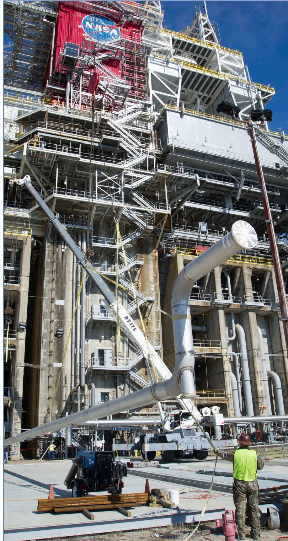
A work crew completes installation of an 18-inch-diameter hydrogen vent line at the B-2 Test Stand at Stennis Space Center early in February. Installation of the vent line, fabricated on site and installed by Syncom Space Services personnel, is part of preparations for testing the flight core stage of NASA's new Space Launch System rocket on the Stennis stand. Testing will involve installing the actual flight stage on the stand and firing all four of its RS-25 engines simultaneously, as during a launch. RS-25 engines burn a mixture of liquid hydrogen and liquid oxygen. During testing, the vent line and attached flare stack are used to bleed and burn off excess liquid hydrogen from vehicle vent and engine bleed lines so it can be released safely into the atmosphere. Work crews earlier moved the hydrogen flare stack from the A-1 Test Stand back to its original B-2 location.
