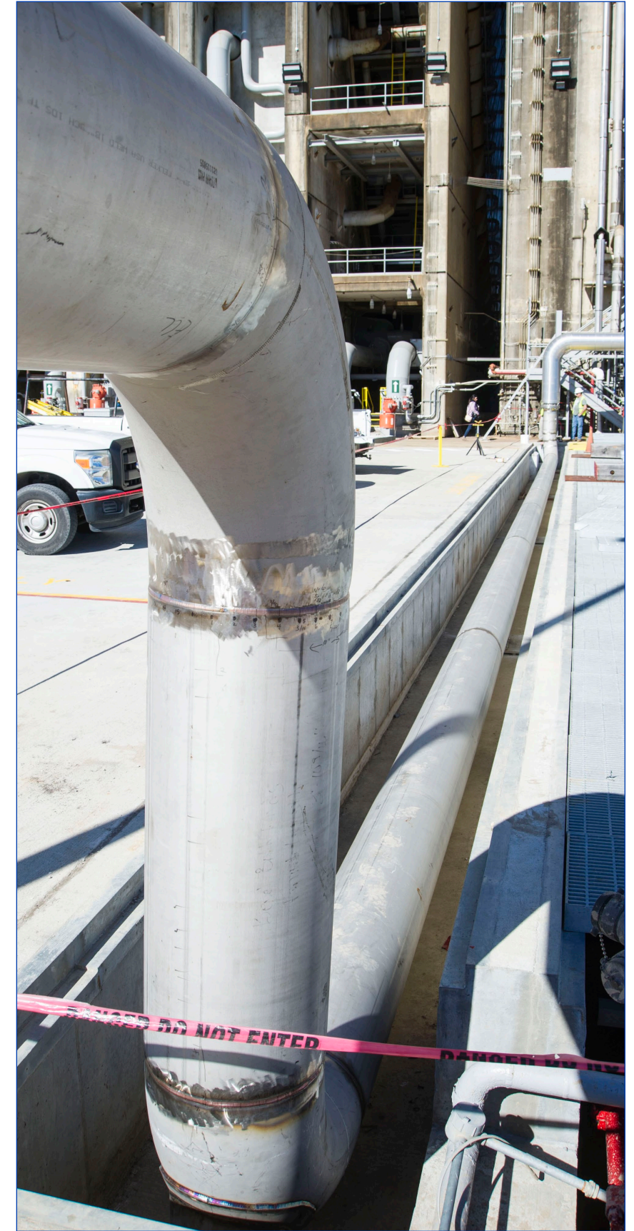
A work crew completes installation of an 18-inch-diameter hydrogen vent line at the B-2 Test Stand at Stennis Space Center early in February. Installation of the vent line, fabricated on site and installed by Syncom Space Services personnel, is part of preparations for testing the flight core stage of NASA's new Space Launch System rocket on the Stennis stand. Testing will involve installing the actual flight stage on the stand and firing all four of its RS-25 engines simultaneously, as during a launch. RS-25 engines burn a mixture of liquid hydrogen and liquid oxygen. During testing, the vent line and attached flare stack are used to bleed and burn off excess liquid hydrogen from vehicle vent and engine bleed lines so it can be released safely into the atmosphere. Work crews earlier moved the hydrogen flare stack from the A-1 Test Stand back to its original B-2 location.
