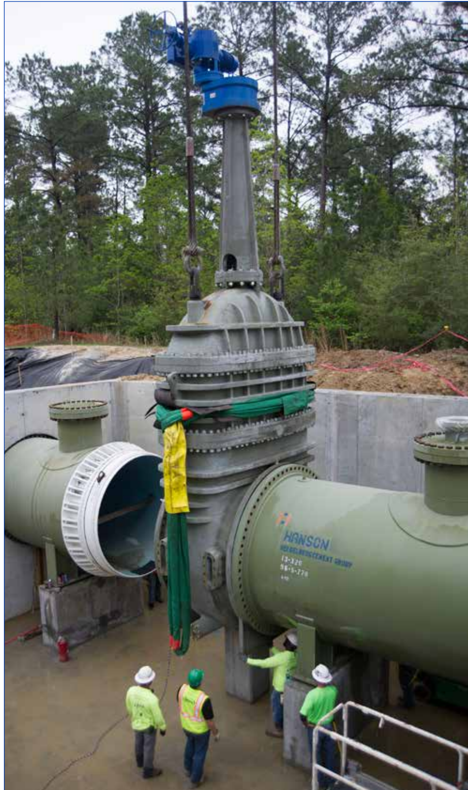
(Top left photo) Stennis Space Center employees install a 96-inch valve March 26 as part of an ongoing project to upgrade the high-pressure industrial water system that serves the site's large rocket engine test stands.
