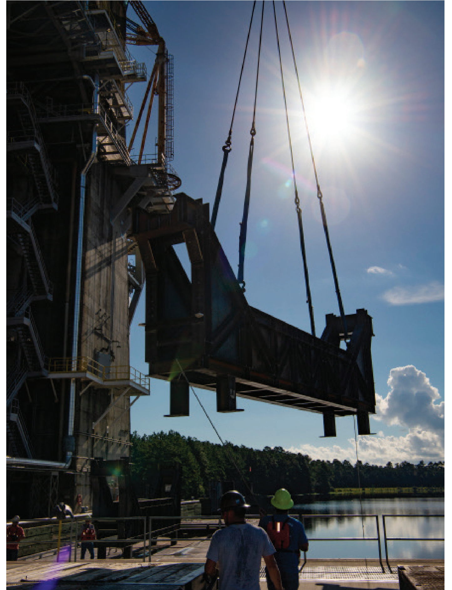
(Top left photo) Launcher's 3D-printed Engine-2 (E-2) rocket engine completes a 5-second hot fire Aug. 20 of its latest thrust chamber assembly (Credit: Launcher / John Kraus Photography). (Right photo) The arrival of two trusses marks the first of several large elements needed to prepare the B-2 Test Stand for Green Run testing of the Exploration Upper Stage unit being built for use on future Space Launch System missions. (Bottom left photo) The spike diffuser is a new design developed and tested at Stennis on the E-3 Test Stand.
