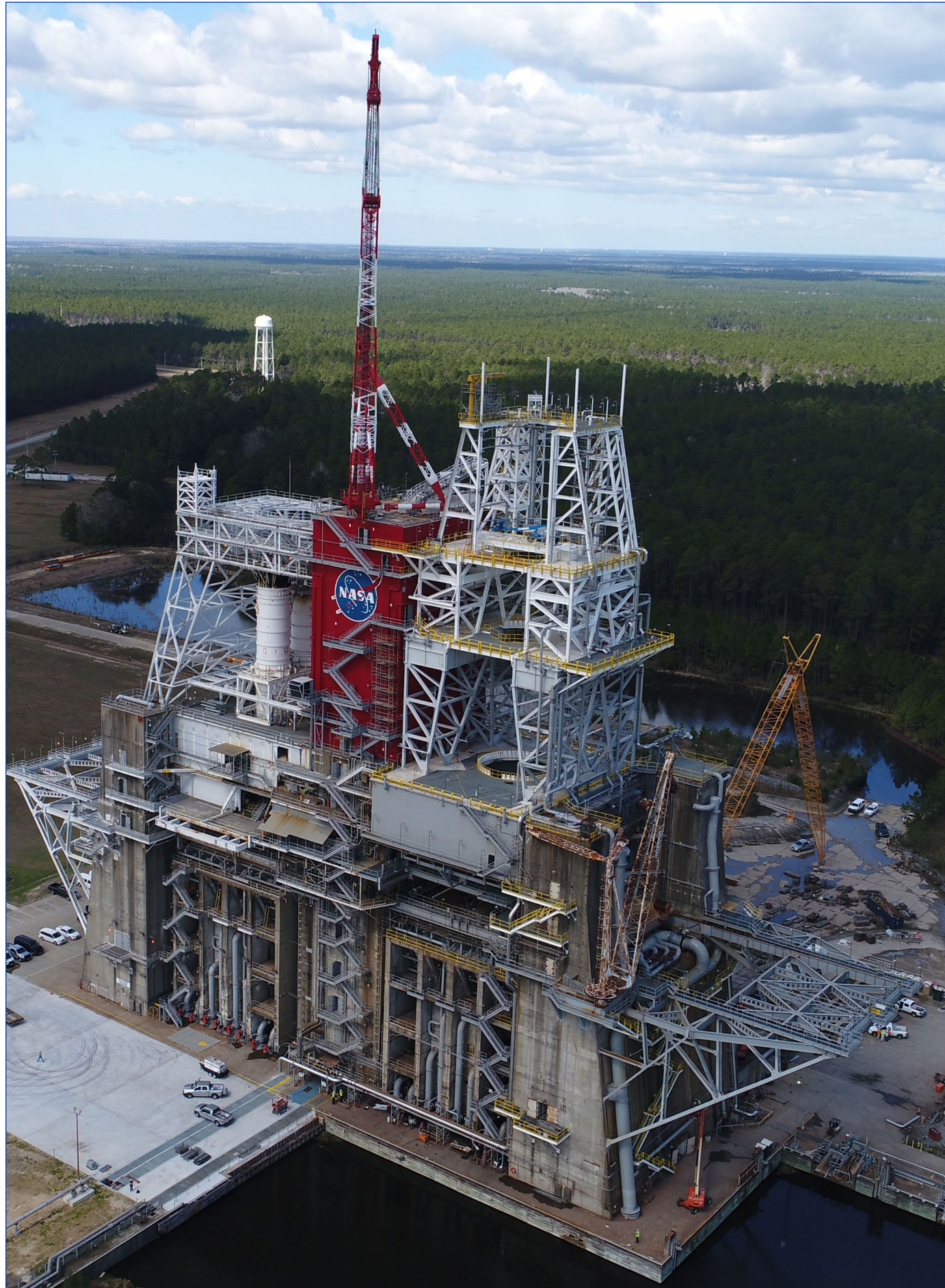
(Left photo) An unmanned drone photo offers an on-high look of the B-1/B-2 Test Stand at Stennis Space Center, highlighting modifications made to enable testing of NASA's new Space Launch System (SLS) core stage. The SLS stage will be tested on the B-2 portion of the stand, shown to the right.
