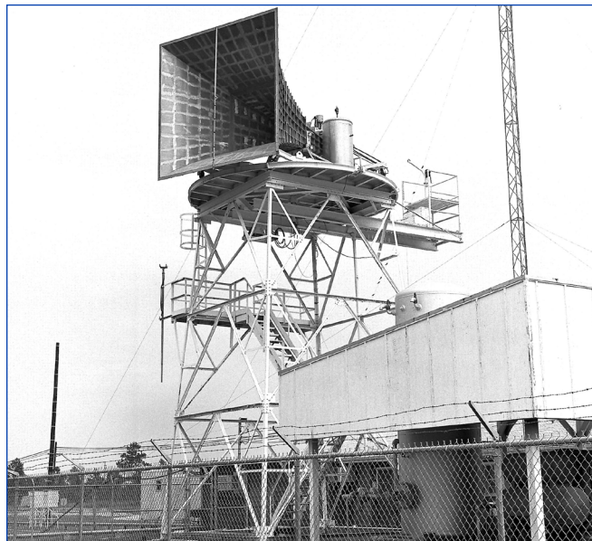
A 1965 photo shows the acoustical air horn used by NASA to conduct noise level studies prior to rocket engine and stage testing at Stennis.
