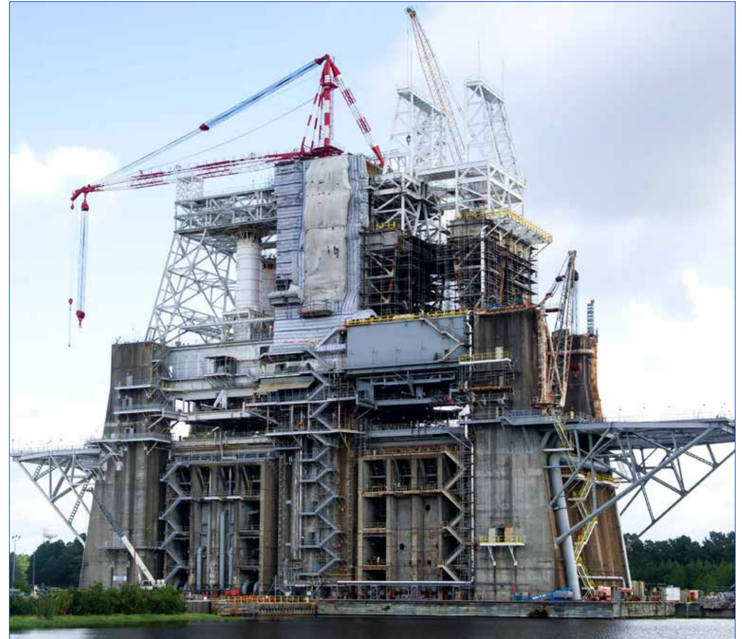
(Above photo) This 2003 image shows the B-1/B-2 Test Stand as it looked before NASA began renovation work to prepare for Space Launch System stage testing. (Right photo) A recent image shows the new profile of the B-1/B-2 Test Stand. The white framework structure on the right is needed to accommodate the large Space Launch System core stage, which will be tested at Stennis prior to a scheduled 2018 flight.
