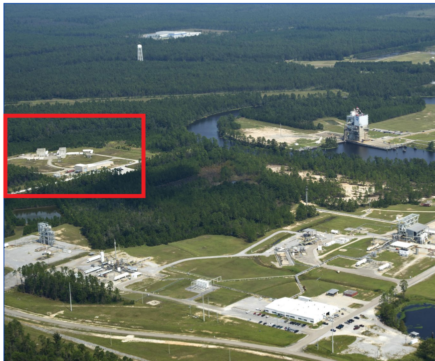
An aerial photos shows the A-1 Test Stand (top right) and the E Test Complex (foreground facilities) at Stennis Space Center. The E-4 test area to be developed by Relativity Space is the small cluster of facilities and unfinished test cells at the top left, indicated by the red square.
