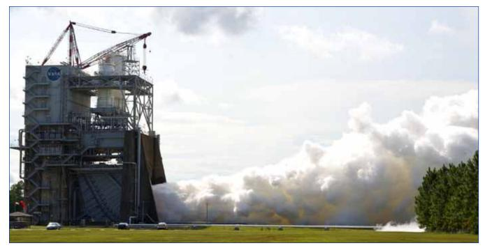
J-2X Engine No. 10002 is test fired for the final time on the A-1 Test Stand at NASA's Stennis Space Center. The 330-second test was the last in a series of gimbal, or pivot, tests on the engine. Following the removal of this engine, the test stand will be modified to begin RS-25 engine testing. J-2X testing has provided valuable data and experience for the team developing the RS-25 engine, which will power the core stage of NASA's new Space Launch System.
