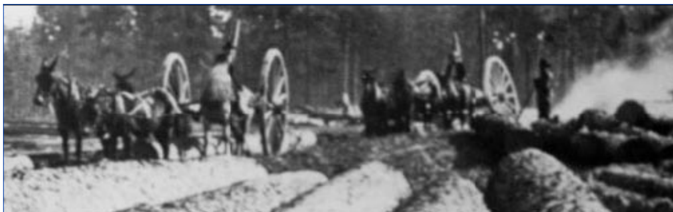
Usan Vaughn invented the famous high-wheeled, wide-tread carrylog (caralog) shown above that made it possible for logging crews to work in wet ground and haul out logs of any size with their sturdy ox teams.
