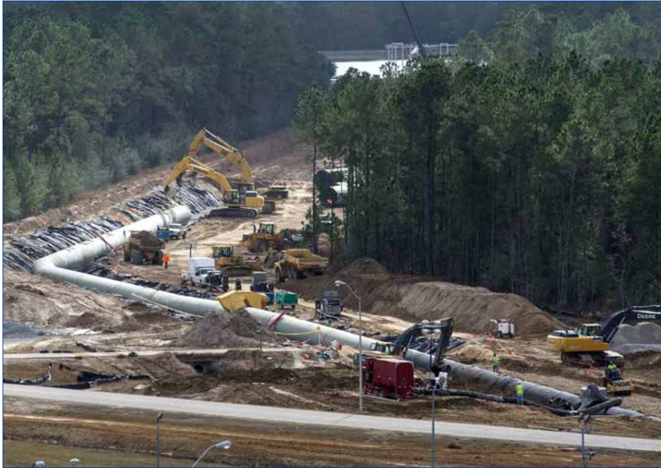
(Above photo) Work progresses on the high-pressure industrial water project at Stennis Space Center. The project involves replacing and upgrading full sections of large piping that provide water to Stennis test stands, a critical need during hotfire testing of rocket engines.
