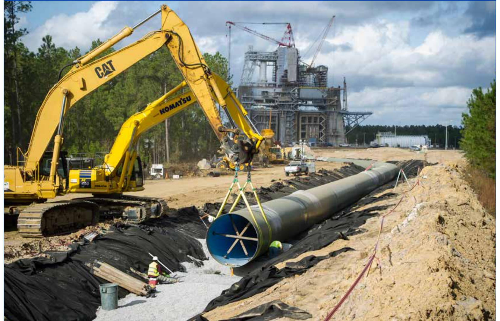
(Above photo) Work progresses on the high-pressure industrial water project at Stennis Space Center. The project involves replacing and upgrading full sections of large piping that provide water to Stennis test stands, a critical need during hotfire testing of rocket engines.
