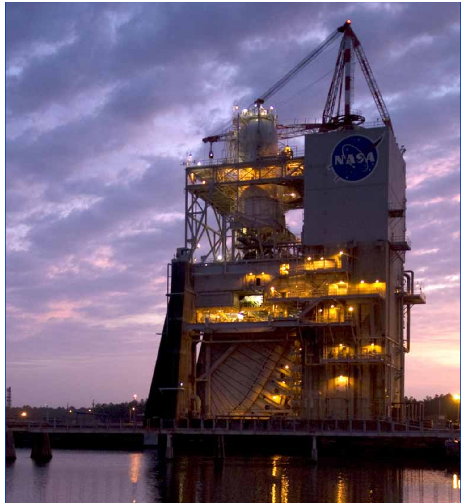
Sunrise frames the historic A-1 Test Stand at Stennis Space Center. Modifications are being made to the stand to enable gimbal testing of the next-generation J-2X rocket engine this summer. NASA engineers recently completed testing of the J-2X powerpack assembly on the stand.
