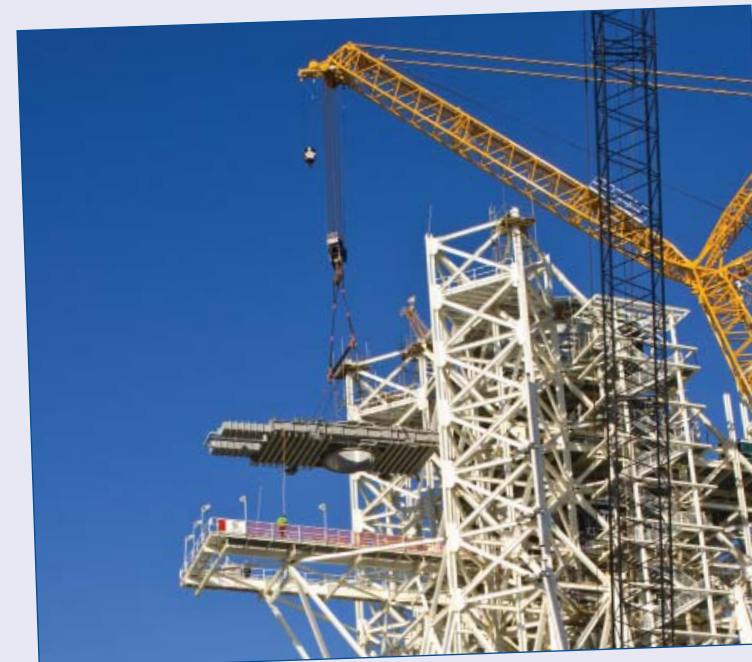
Construction of the A-3 Test Stand at Stennis Space Center featured both large-crane operations and small-scale detail work in 2011. (Clockwise, from top left) The stand as it appeared at the start of 2011. A welder works on supporting structures on the stand. A large crane lifts the test cell dome into place, marking a major "topping out" milestone in April 2011. A test cell isolation valve is installed on the new high-altitude simulation stand. Stennis employees prepare the A-3 Test Stand thrust measurement system for placement.
