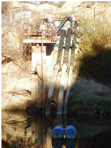
G-21. R2A Pond. R2A Pond Pump intake and piping for water transfers to and from Silvernale Pond. January 5, 2012
