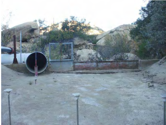
G-17. R2A Pond. Culvert and gated weir from R2A Pond. January 5, 2012
