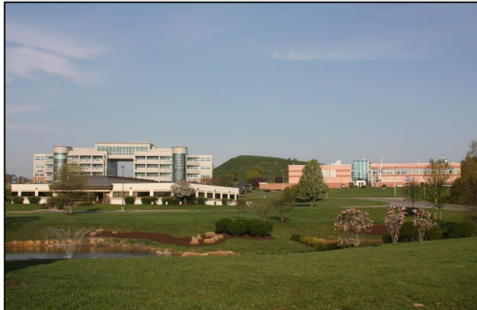
Exhibit 3-12. GSFC – Katherine Johnson Independent Verification and Validation Facility
