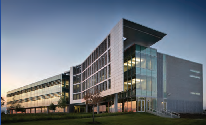
Building 20, LEED Office Facility for Transition, is one of JSC's six completed LEED certified buildings and was the first NASA building to earn the Platinum certification. This building and the other LEED buildings incorporate energy and water conservation techniques, daylighting, renewable materials and other sustainable characteristics in their design and construction.
