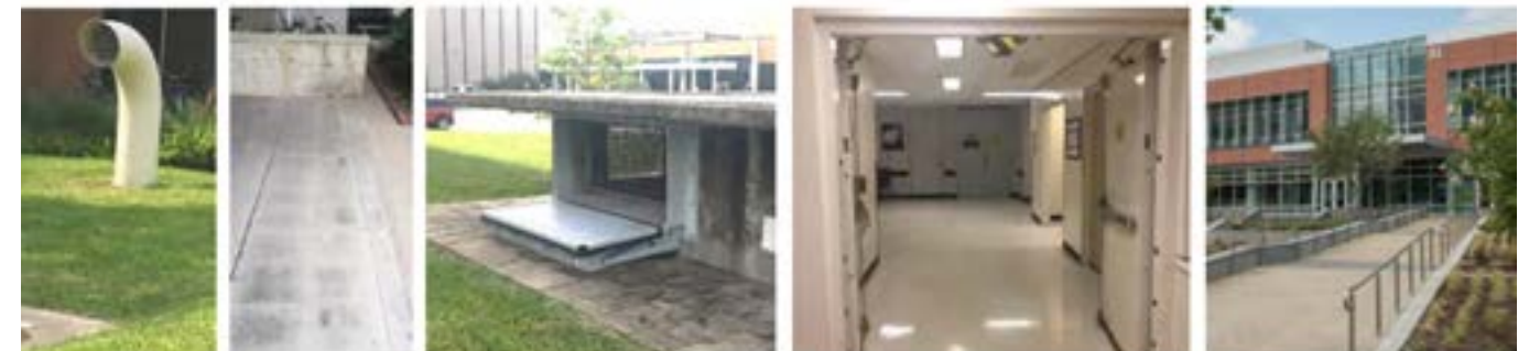
Raised tunnel air intake
