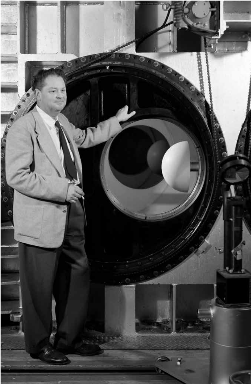
Figure 2.6. H. Julian Allen stands at the observation window of the 8-by-7-foot test section of the Ames Unitary Plan Wind Tunnel, December 1957. A blunt shape, or body, sits inside the test section.
