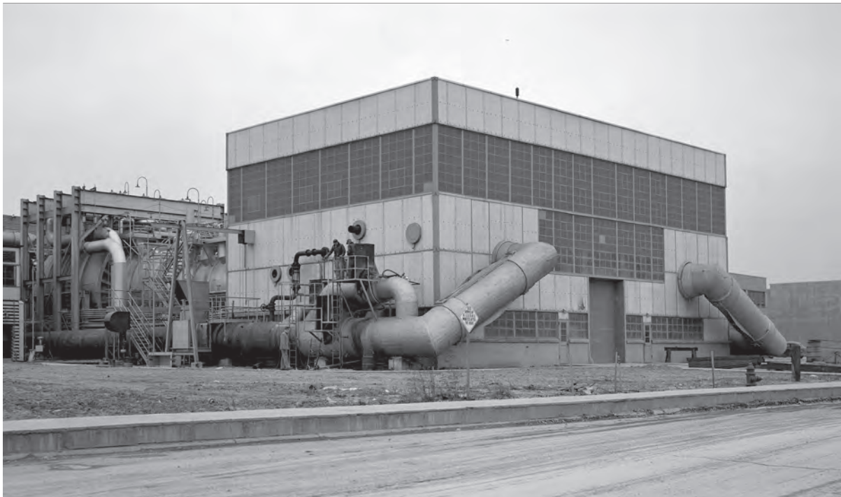
Image 55: After passing through temperature-adjusting equipment, the combustion airflow was pumped through a pipe to one of the test chambers on the second floor of the Shop and Access Building, seen here on 3 February 1953. In 1957 a two-story shop section was added to the front of the building. The pipes remained but were not visible on the exterior. (NASA C-1953-31941)
