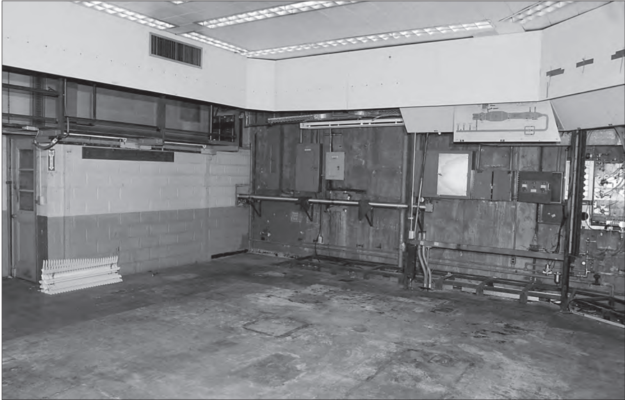
Image 154: Cannibalized control room for PSL No. 1 and 2 on 9 September 2008. The control panels, data systems, and equipment have been removed. The only indication of the room's original function is the combustion air system indicator board hanging on the far wall. (NASA C-2008-04125)
