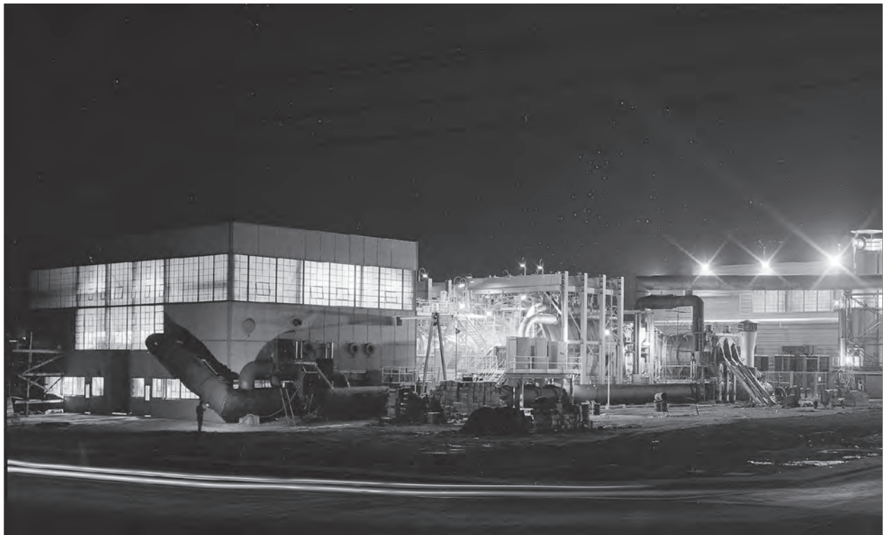
Image 156: The PSL emerging in September 1952 as the nation's premier engine testing facility. (NASA C-1952-30764)
