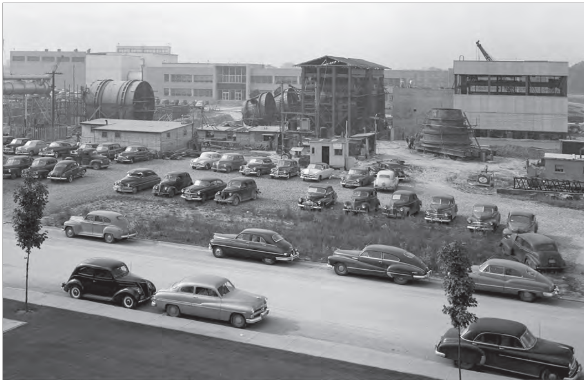
Image 25: This late September 1950 photograph shows the framework for the two primary coolers for the altitude exhaust near the center of the photograph. The Shop and Access Building is being built to the right, and excavation for the Equipment Building has begun in the background to the left. (NASA C-2009-00184)
