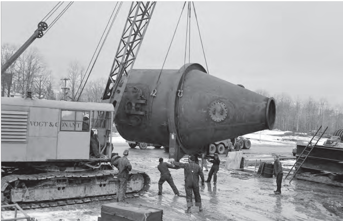
Image 27: The inlet section of one of the PSL altitude chambers is unloaded from a flatbed at the construction site on 5 January 1951. Air would enter the tank through an opening on the right side during operation. (NASA C-2009-00171)
