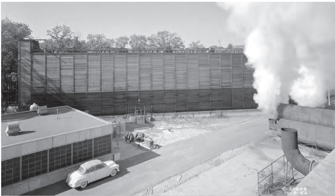
Image 69: The cooling water for the primary and secondary coolers was circulated by the Circulating Water Pump House located across the street. The pump house, seen here in the foreground on 8 October 1952, contained the large water pumps and water-softening units. The water carrying the heat was sprayed down into the large, adjacent cooling tower. Roof fans in the wooden tower ceiling exhausted the hot air out as the water was diffused into the pools at the bottom. (NASA C-1952-30938)
