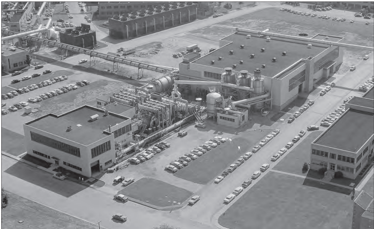
Image 2: The PSL No. 1 and 2 facility viewed from the west on 9 June 1959. The Shop and Access Building containing the two test chambers is to the left, and the larger Equipment Building containing the exhausters and compressors is behind and to the right. (NASA C-1959-50861)
