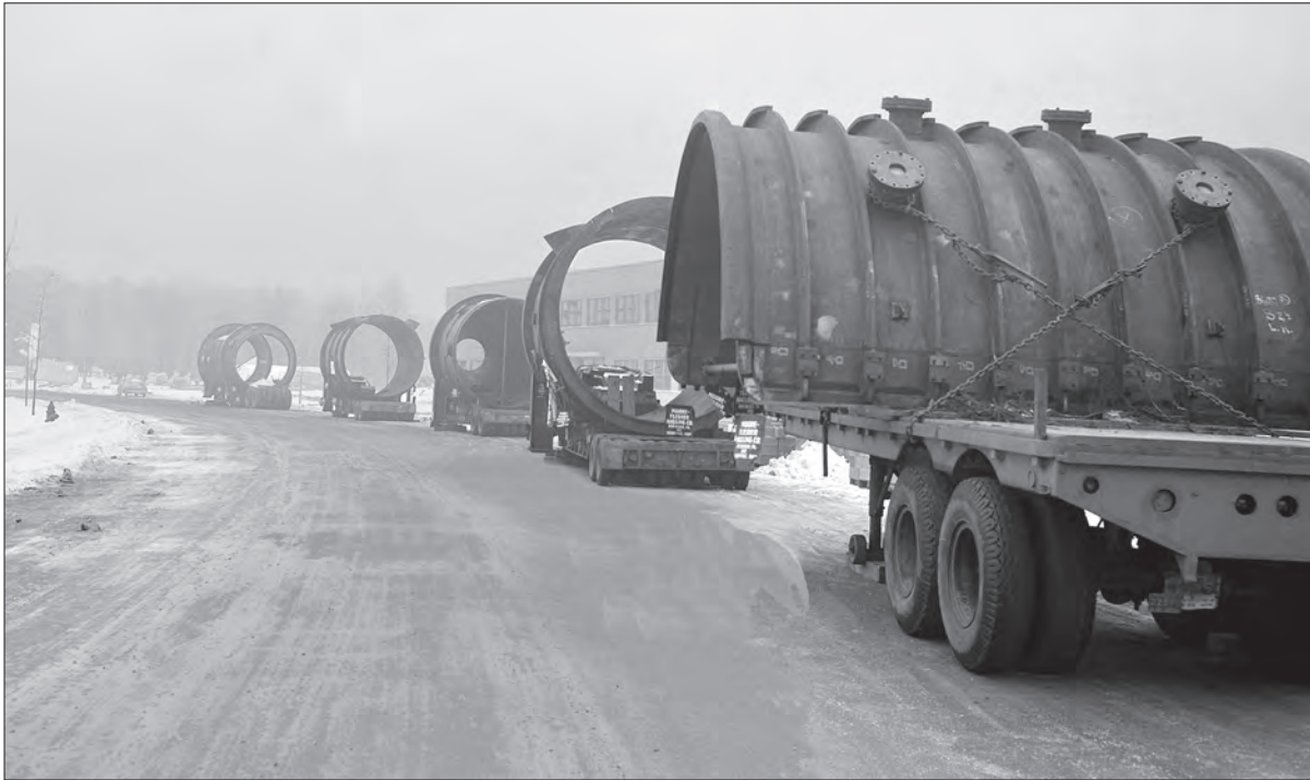
Image 26: A caravan of large steel castings manufactured by the Henry Pratt Company arrived on 5 January 1951 for the PSL altitude chambers. The massive pieces were delivered to the area by rail and then loaded on a series of flatbed trucks that transported them to Lewis. The nearest vehicle has one of the clamshell access hatches. (C-2009-00173)
