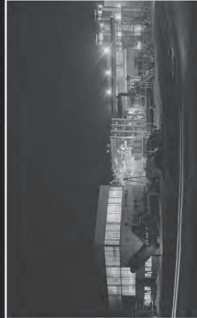
PSL No. 1 and 2 was the National Advisory Committee for Aeronautics and National Aeronautics and Space Administration's largest propulsion systems laboratory in the 1950s and 1960s at simulator altitudes. PSL was built in the late 1940s to expand upon the Wind Tunnel. The facility originally contained two altitude chambers with 14-ft-diameter and 24-ft-long test cells. The test cells were used to test turbojet, turbo-propeller, and turbofan engines. The test cells were used to test the air for altitude simulation and remove the hot gases from the engine. The engine test cell was used to test the engine.
