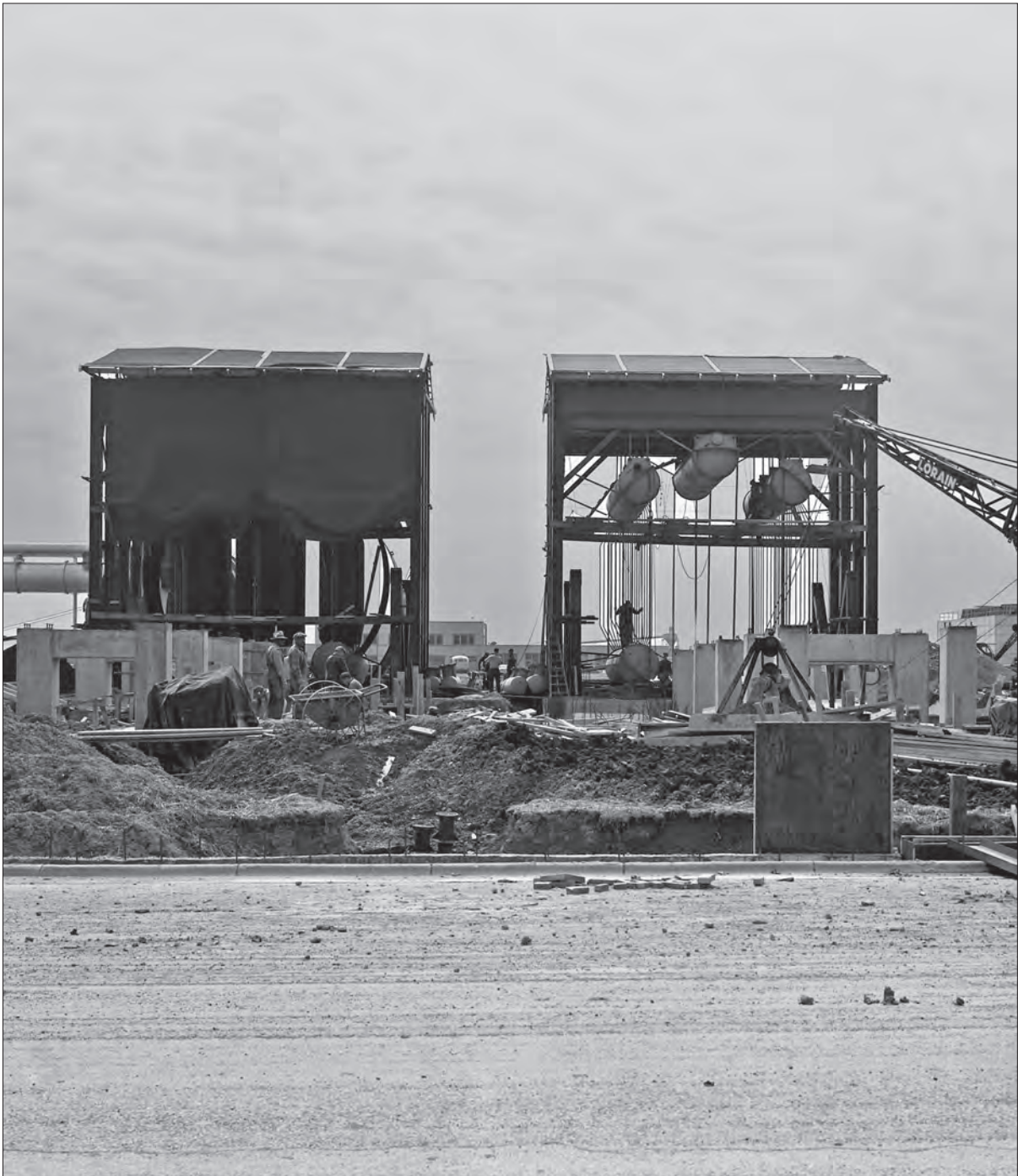
Image 18: These two stands were erected to hold PSL's two primary coolers on 26 April 1950. Construction at the site had been under way for approximately six months at this point. (NASA C-2009-00175)
