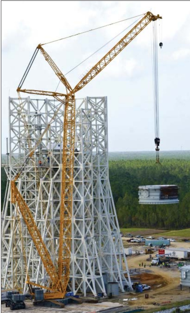
Work on the A-3 Test Stand at Stennis Space Center took milestone strides forward in July with delivery and installation of the first-stage steam ejector and parts of the test cell. Work on the stand began in 2007. When activated in 2012, it will allow operators to test rocket engines at simulated altitudes of 100,000 feet, a critical feature for next-generation engines that will take humans beyond low-Earth orbit once more. (Above photo) A section of the A-3 test cell is lifted onto the structural steel frame for installation. (Top right photo) A barge negotiates the Stennis locks for delivery of A-3 Test Stand components July 15. (Middle right photo) Workers prepare the first-stage steam ejector for lifting and installation onto the A-3 Test Stand frame. (Bottom right photo) A component of the A-3 test cell sits on the stand's structural steel frame after installation.
