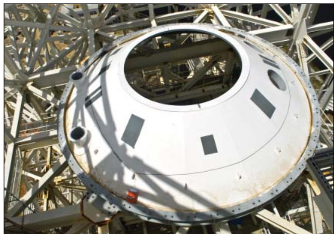
Work on the A-3 Test Stand at Stennis Space Center took milestone strides forward in July with delivery and installation of the first-stage steam ejector and parts of the test cell. Work on the stand began in 2007. When activated in 2012, it will allow operators to test rocket engines at simulated altitudes of 100,000 feet, a critical feature for next-generation engines that will take humans beyond low-Earth orbit once more. (Above photo) A section of the A-3 test cell is lifted onto the structural steel frame for installation. (Top right photo) A barge negotiates the Stennis locks for delivery of A-3 Test Stand components July 15. (Middle right photo) Workers prepare the first-stage steam ejector for lifting and installation onto the A-3 Test Stand frame. (Bottom right photo) A component of the A-3 test cell sits on the stand's structural steel frame after installation.
