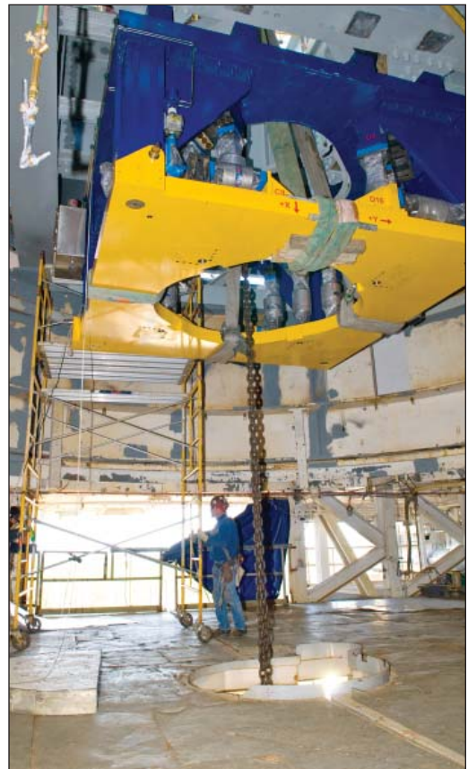
(Bottom right photo) Stennis employees complete installation of the new TMS on the A-1 Test Stand.
