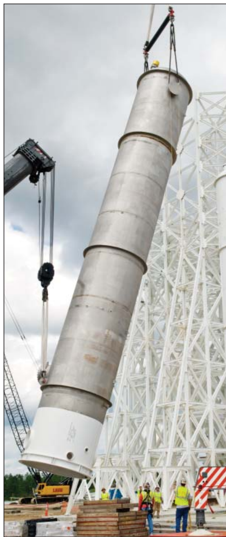
and liquid oxygen (above, right) tanks recently were delivered and installed at the A-3 Test Stand under construction at Stennis Space Center.
