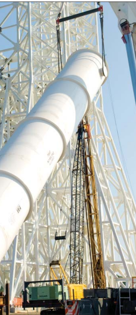
and liquid oxygen (above, right) tanks recently were delivered and installed at the A-3 Test Stand under construction at Stennis Space Center.
