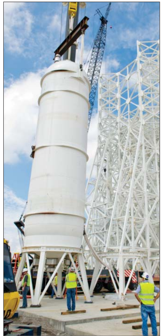
and liquid oxygen (above, right) tanks recently were delivered and installed at the A-3 Test Stand under construction at Stennis Space Center.
