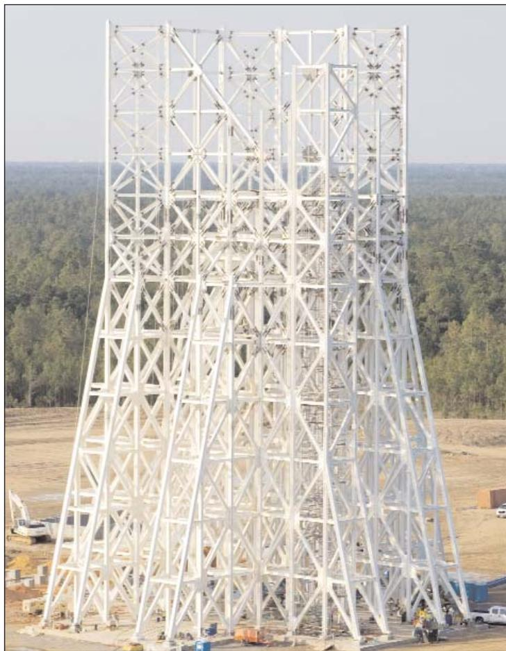
Workers at Stennis Space Center continue construction of a new 300-foot stand that will be used to test engines that will help humans go back to the moon.
