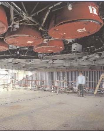
(Left photo) Stennis Space Center workers monitor the installation of the S-II-1 Saturn stage on the A-2 Test Stand in August 1966.
