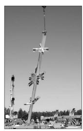
One of the first pieces of fabricated steel is lifted into place in late October at the A-3 Test Stand site.
