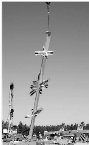
One of the first pieces of fabricated steel is lifted into place in late October at the A-3 Test Stand site.
