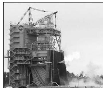
Smoke and flames bear evidence of the success of an April test of the J-2X power pack 1A at the A-1 Test Stand.
