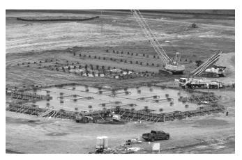
**FINISHED PRODUCT** – With concrete in place Dec. 9, the 160-foot-by-160-foot A-3 base takes shape. The foundation remained under plastic cover for about seven days, and will be allowed to cure undisturbed over the next several weeks. The mix of the material is designed to bear a load of 4,000 pounds per square inch when hardened.
