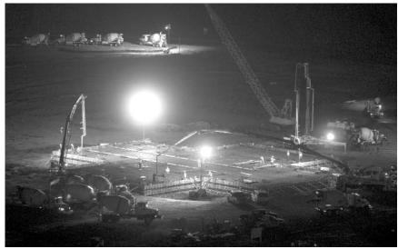
**LIGHTING THE WAY** – Floodlamps illuminate the site of Stennis Space Center's future A-3 Test Stand as concrete trucks jockey for position to deliver their product. Over a 14-hour period beginning at 6 p.m. Dec. 8, more than 400 trucks delivered 3,365 cubic yards of concrete for the stand's foundation. The task was scheduled at night to ensure an uninterrupted traffic flow on local and on-site roads.
