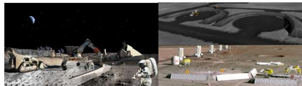
Civil engineering, infrastructure emplacement and structure construction from *in situ* derived materials ➤ Radiation shields, landing pads, roads, berms, habitats, etc.
