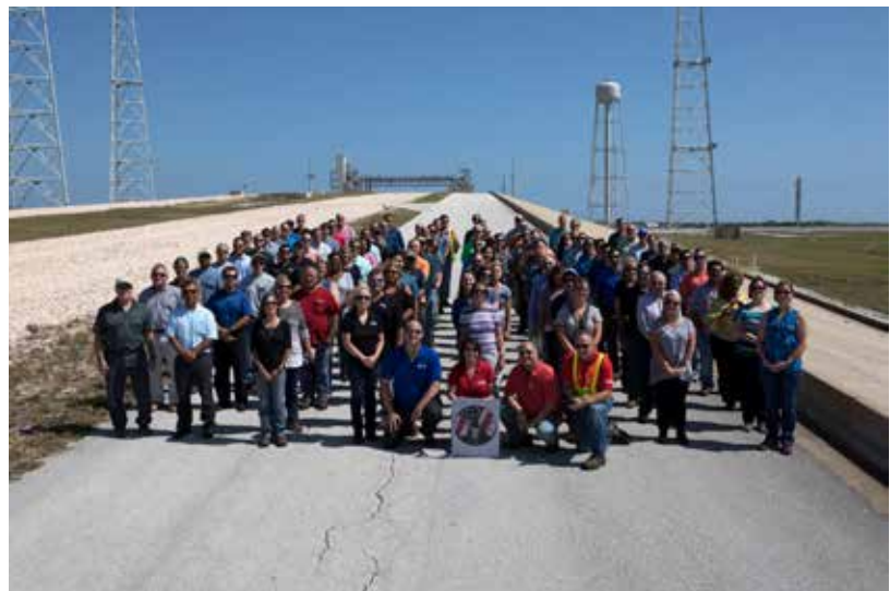
Launch Complex 39B current and past NASA and contractor workers gathered at Pad B to mark the 50th anniversary of the launch complex. Upgrades to the surface of Pad B, as well as the systems below and surrounding the pad will support the new processing and launch requirements for NASA's Space Launch System (SLS) and the Orion spacecraft for deep space missions, including to the Moon, Mars and beyond. The modifications and improvements to processing and launch facilities will support Kennedy as a multi-user spaceport for government and commercial launches for years to come.
