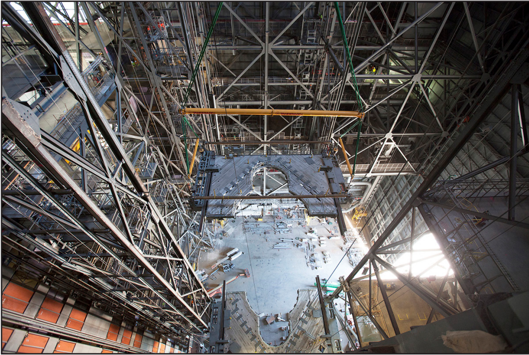
A 250-ton crane is used to lower the second half of the K-level work platforms into High Bay 3 on March 7. The platform was secured about 86 feet above the VAB floor, on tower E of the high bay. The K work platforms will provide access to the SLS core stage and solid rocket boosters during processing and stacking operations on the mobile launcher. Photo credit: NASA/Dimitri Gerondidakis
