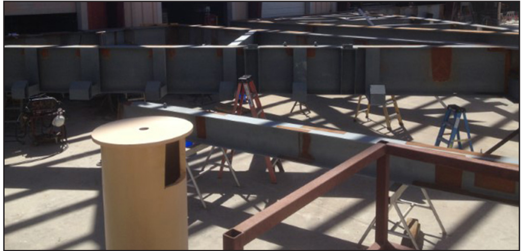
Preliminary assembly of a platform for High Bay 3 is in progress in September at Sauer Inc. in Oak Hill, Florida.
