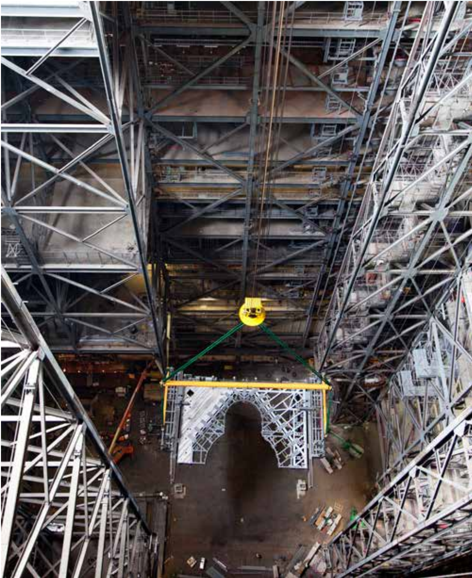
A view from high above in the Vehicle Assembly Building at Kennedy Space Center on Dec. 22, 2015, shows a 325-ton crane lifting the first half of the K-level work platforms for installation in High Bay 3. The K work platforms will provide access to NASA's Space Launch System core stage and solid rocket boosters during processing and stacking operations on the mobile launcher.
