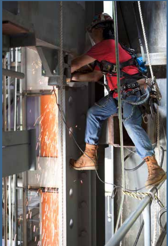
A tethered construction worker wearing safety gear works on one of the bolts during installation of the second half of the J-level work platforms April 15, 2016, for NASA's a Launch System rocket in High Bay 3 inside the Vehicle Assembly Building at Kennedy Space Center. The platform was installed about 112 feet above the floor, or nearly 11 stories high, inside the high bay.
