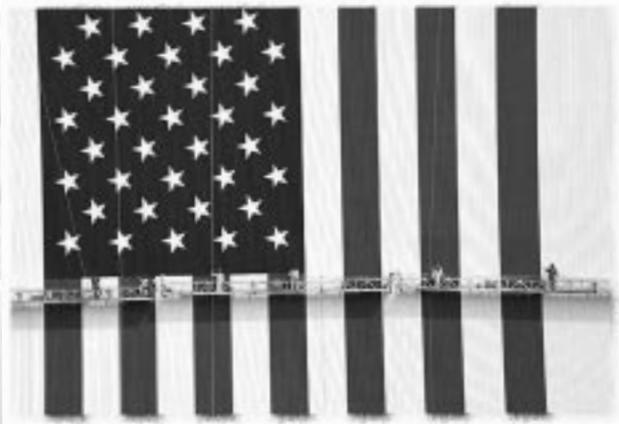
The Vehicle Assembly Building (VAB), the Center's largest and most visible icon, sustained a makeover. KSC workers used 700 gallons of paint to refurbish one of the world's largest structures in preparation for the center's 40th anniversary, replacing a bicentennial symbol with the round, blue NASA insignia affectionately known as the "meatball."
