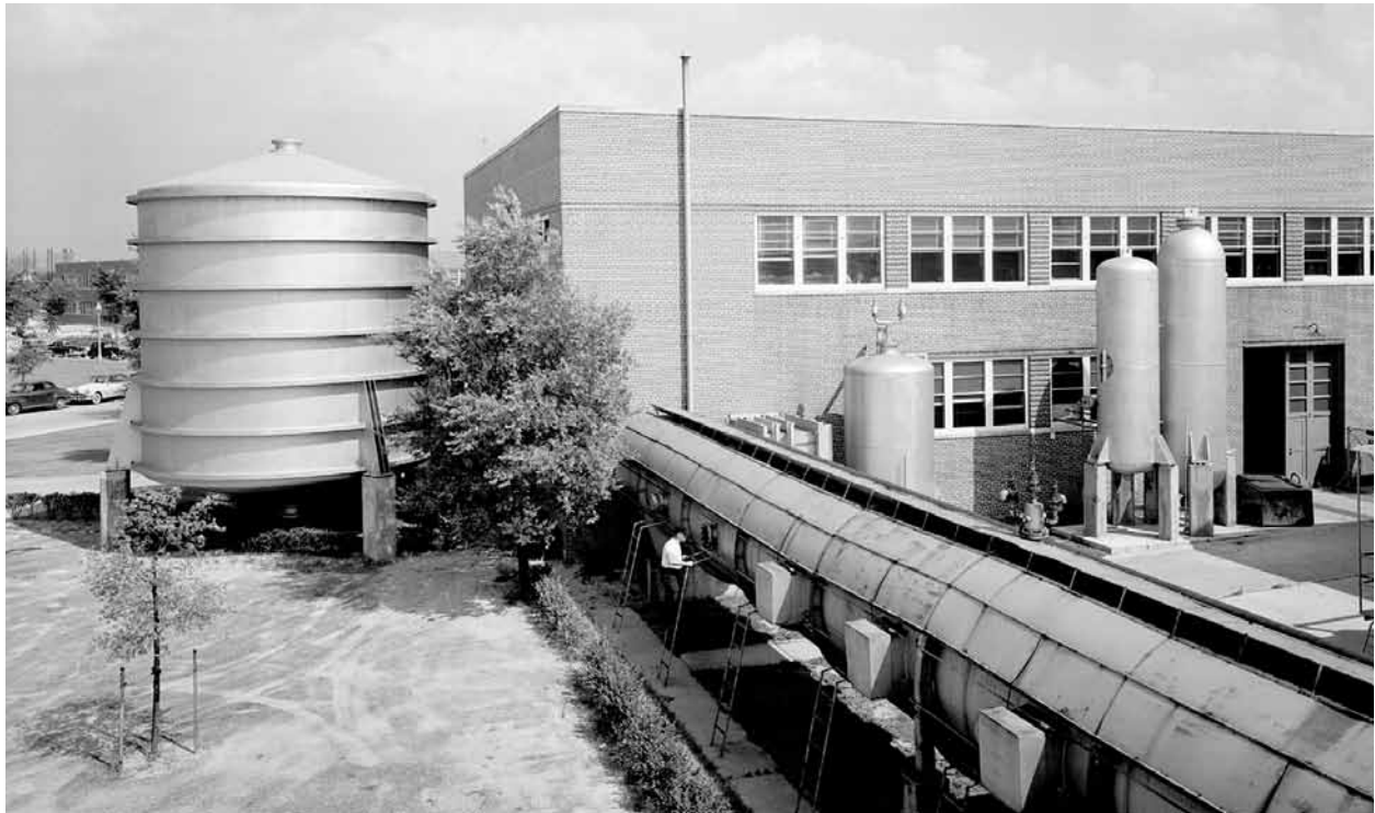
View of the Physical Research Laboratory at Langley in 1949 showing the ill-fated Langley Free-Flight Facility in the foreground. The 100-foot-long, 8-foot-diameter facility was equipped with viewing windows but suffered poor flow characteristics during model flights and was closed before meaningful research results were obtained.
