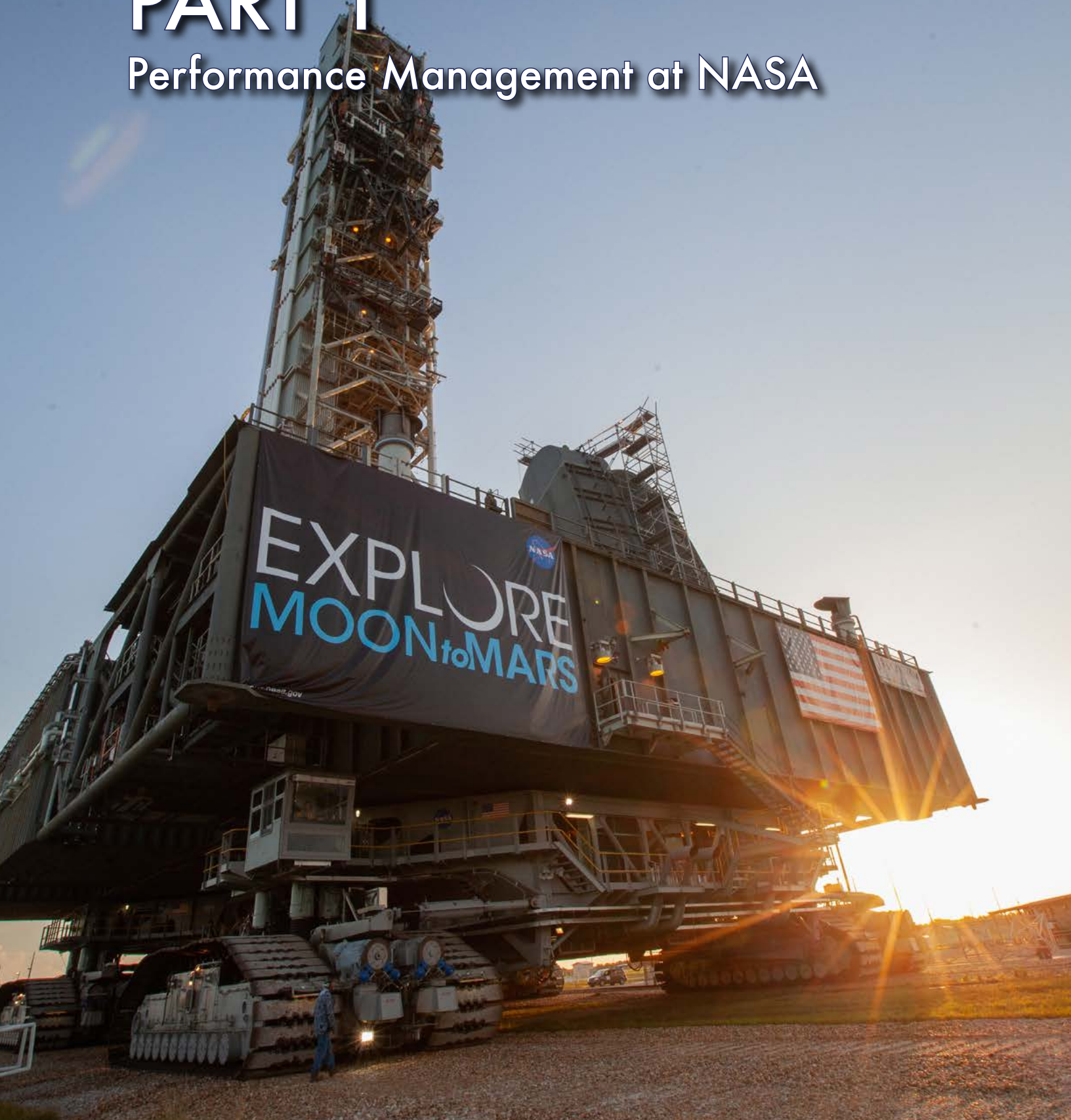
The Sun rises as NASA's crawler-transporter 2, carrying the mobile launcher, arrives at the NASA Kennedy Space Center's Launch Complex 39B on June 28, 2019. The mobile launcher underwent final testing and checkout during the summer in preparation for the launch of Artemis 1. Photo credit: NASA/Ben Smegelsky
