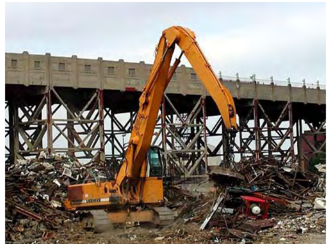
Magnetic cranes are used to lift heavy loads of material containing iron.
