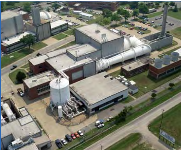
The National Transonic Facility is a modern-day wind tunnel at NASA's Langley Research Center.
