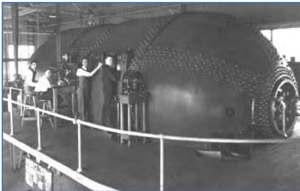
Langley's Variable Density Tunnel could predict how aircraft would perform under flight conditions (1922).
