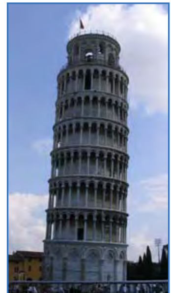
Leaning Tower of Pisa
