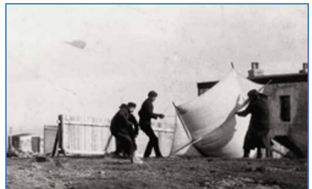
Photograph of Marconi and associates raising the receiving antenna by kite at St. John's, Newfoundland in December, 1901.
