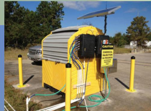
A solar-powered In Situ Chemical Oxidation control system at Stennis Space Center.
