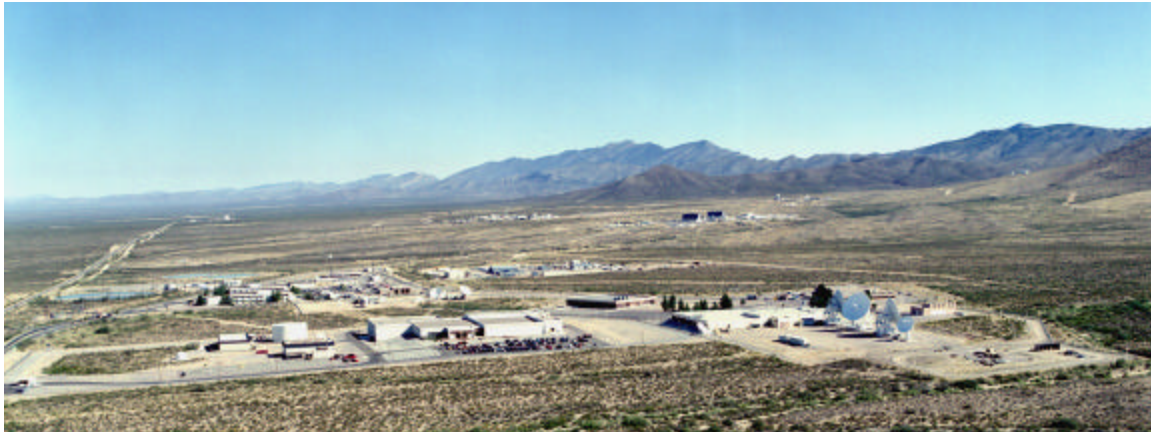
Aerial view of White Sands Test Facility northeast of Las Cruces, New Mexico
