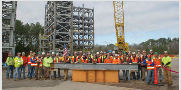
Prime contractor Brasfield & Gorrie of Birmingham, Alabama, and several of its subcontractors are constructing Test Stand 4697 and Test Stand 4693 .
