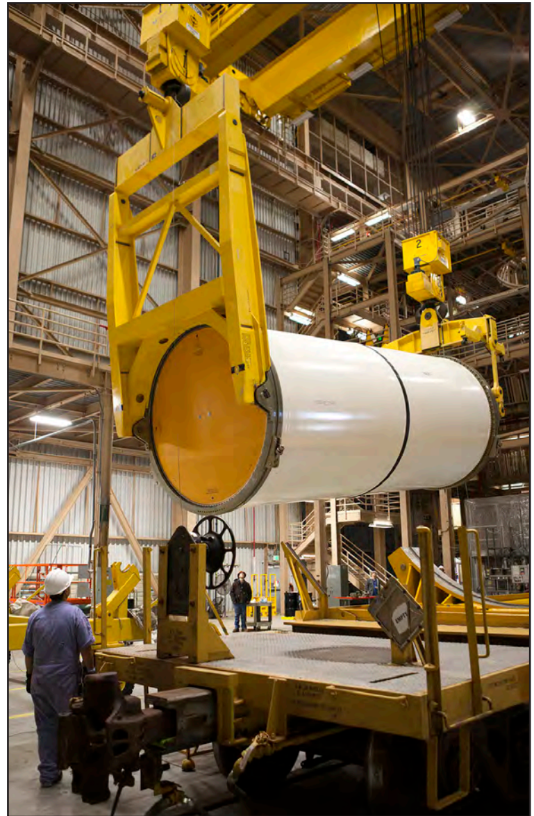
Inside the Rotation, Processing and Surge Facility high bay at NASA's Kennedy Space Center in Florida, engineers and technicians with Jacobs Engineering on the Test and Operations Support Contract monitor the progress Feb. 25 as two cranes are used in tandem to lift the first of two pathfinders, or test versions, of solid rocket booster segments for NASA's SLS rocket. Photo credit: NASA/Ben Smegelsky
