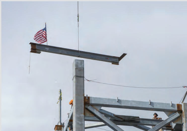
The beam is positioned in place to "top out" Test Stand 4697.
