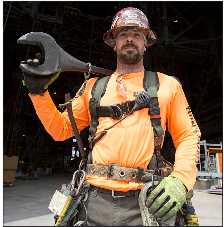
Allen List, an iron and rig foreman with S&R Enterprises of Harrisburg, Pennsylvania, holds a nearly-four-foot-long, 50-pound wrench that he uses to tighten bolts during installation of the large work platforms inside VAB High Bay 3. S&R is a subcontractor to VAB general contractor Hensel Phelps. Photo credit: NASA/Ben Smegelsky
