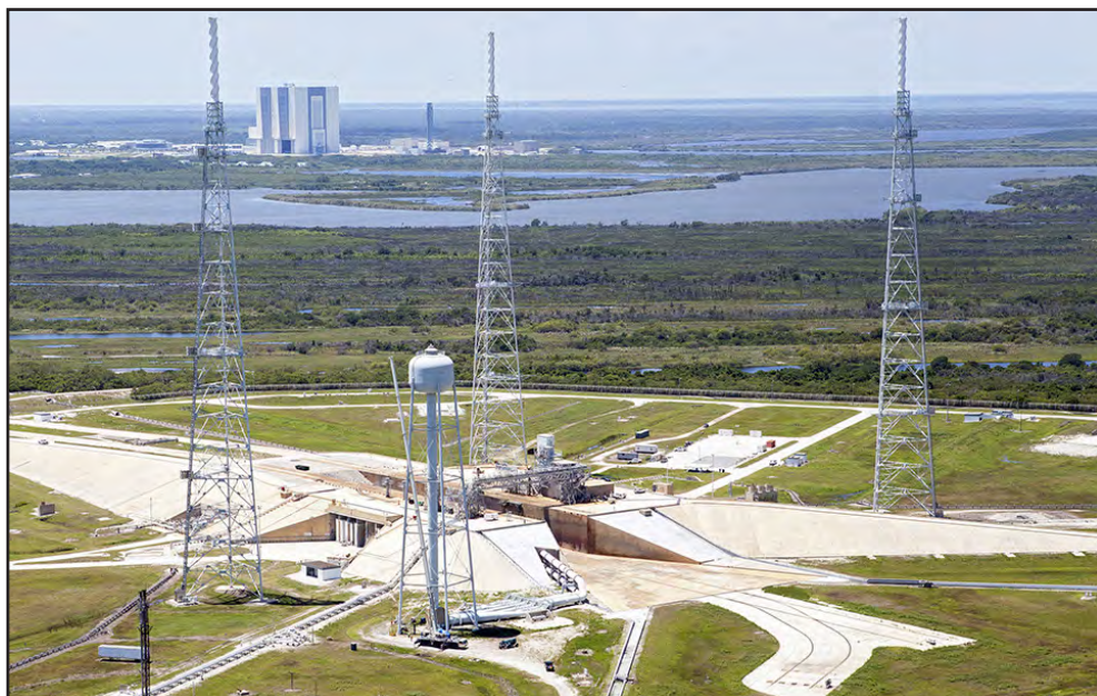
An aerial view of Launch Pad 39B with the Vehicle Assembly Building in the background.
