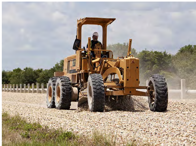
A road grader resurfaces a section of the crawlerway leading from the Vehicle Assembly Building to the launch pads.
