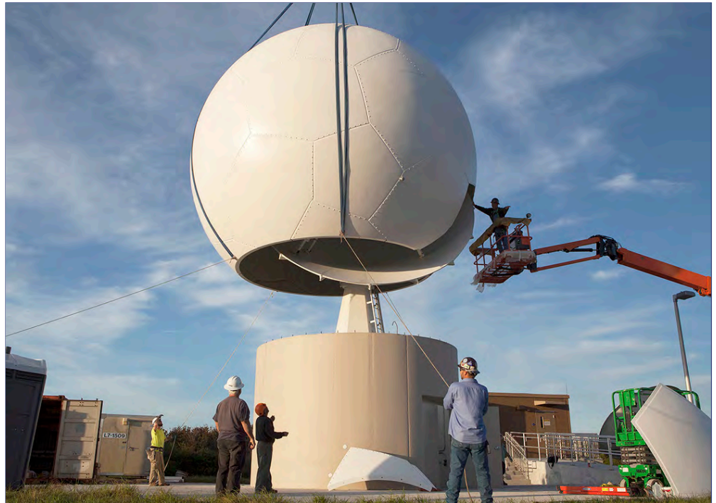
A crane lowers a radome Dec. 10 to cover an S-band antenna at Kennedy Space Center. The antenna is designed to provide a crucial tracking capability following liftoff of NASA's Space Launch System rocket. A radome is a weatherproof structural enclosure designed to protect an antenna or radar system and is constructed of material that interferes minimally with the electromagnetic signal transmitted or received. The S-band portion of the microwave spectrum combines voice, television, telemetry, command, tracking and ranging into a single system. Photo credit: NASA/Dimitri Gerondidakis
