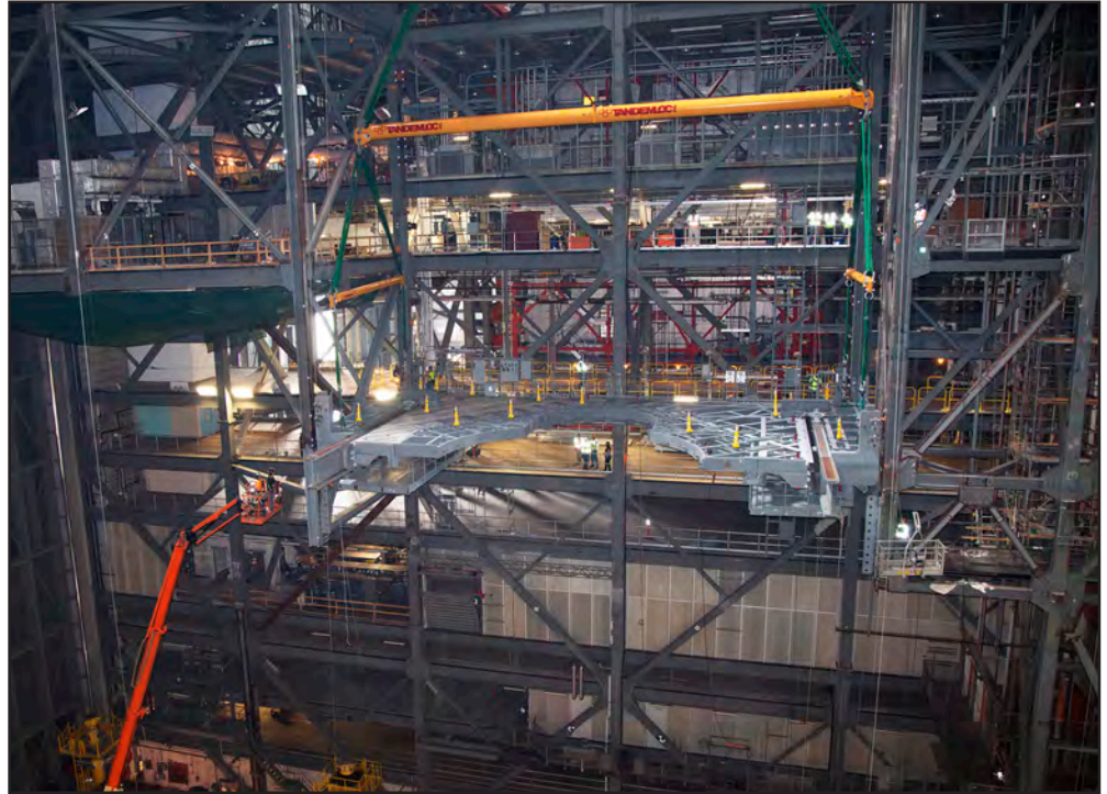
Inside the Vehicle Assembly Building at Kennedy Space Center, a 325-ton crane lifts the first half of the K-level work platforms up for installation in High Bay 3 on Dec. 22. The platform was secured into position on tower E, about 86 feet above the floor. Photo credit: NASA/Ben Smegelsky
