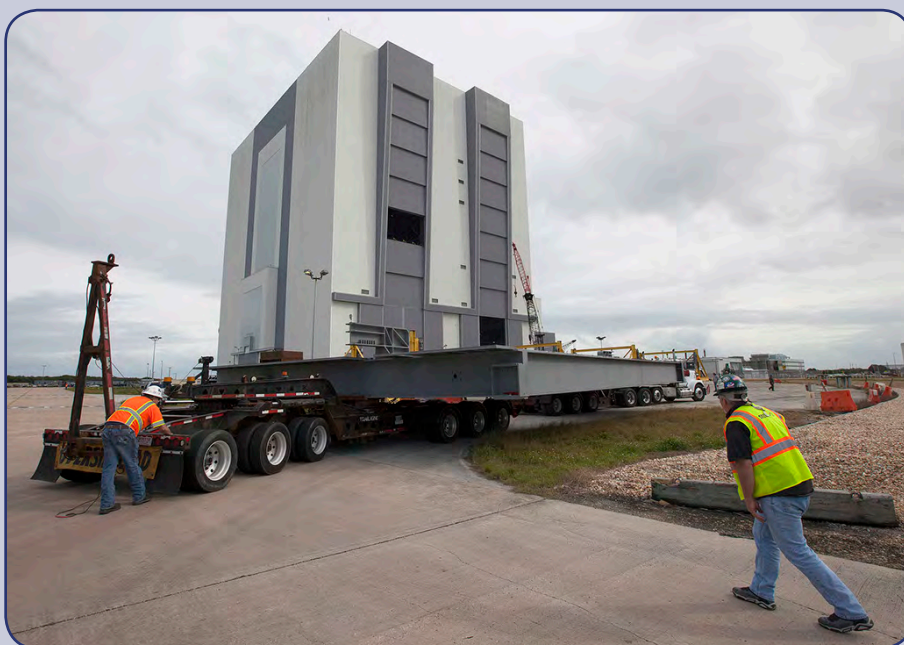
Technicians assist as an oversized, heavy transport trailer, carrying the first half of the "G" level work platforms, proceeds toward the west side parking area of the Vehicle Assembly Building at NASA's Kennedy Space Center in Florida. The platform was transported Jan. 6, from Sauer Co. in Oak Hill, Florida. The Ground Systems Development and Operations Program is overseeing upgrades and modifications to High Bay 3 to support processing of NASA's Space Launch System and Orion spacecraft, and other exploration vehicles. Photo credit: NASA/Ben Smegelsky
