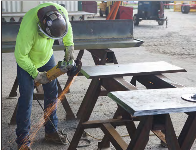
Modifications continued May 28, 2014, on the Mobile Launcher, or ML, at the Mobile Launcher Park Site at Kennedy Space Center. A construction worker trims a section of a steel wall. The ML is being modified and strengthened to accommodate the weight, size and thrust at launch of NASA's Space Launch System and Orion spacecraft.
