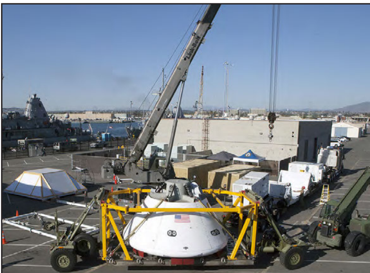
Workers simulated moving the Orion boilerplate test vehicle in place for lifting into the crew module transportation fixture May 14, 2014, at the Mole Pier at Naval Base San Diego in California.
