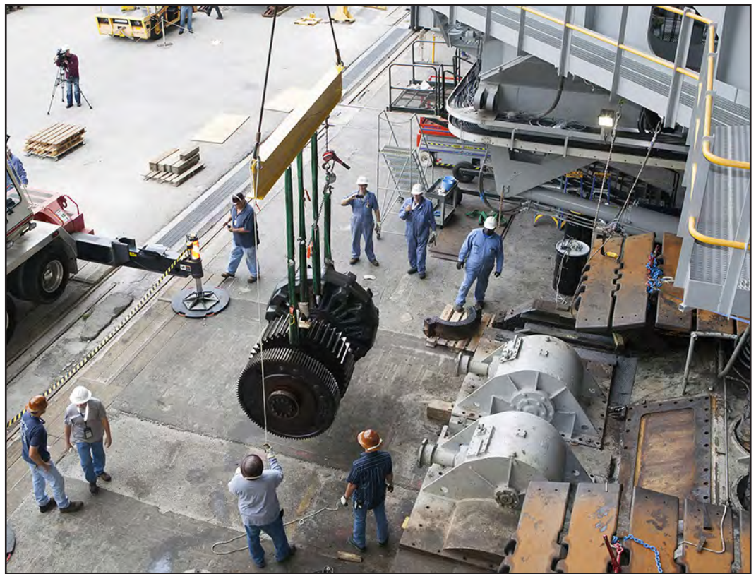
Inside the Vehicle Assembly Building at Kennedy Space Center, ground support technicians monitored the progress as an overhead crane lifted a sprocket shaft assembly away from the crawler-transporter 2 on April 17. A section of the treads were removed to allow access to the sprocket assemblies.
