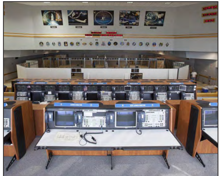
Construction workers have installed the framing and some of the inner walls inside Firing Room 4 in the Launch Control Center.
