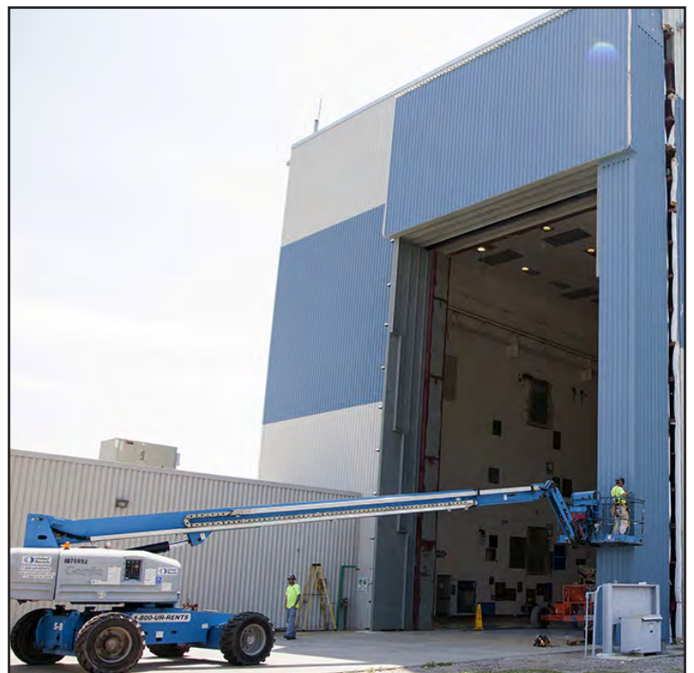
Modifications continued on the Multi-Payload Processing Facility at Kennedy Space Center. The high bay entrance was recently enlarged and a new door installed. Construction workers are installing new siding around the entrance. The extensive upgrades and modernizations will support processing of Orion spacecraft for NASA's exploration missions. The 19,647-square-foot building, originally constructed in 1995, primarily will be used for Orion hypergolic fueling, ammonia servicing and high-pressure gas servicing and checkout before being transported to the Vehicle Assembly Building for integration with the Space Launch System.
