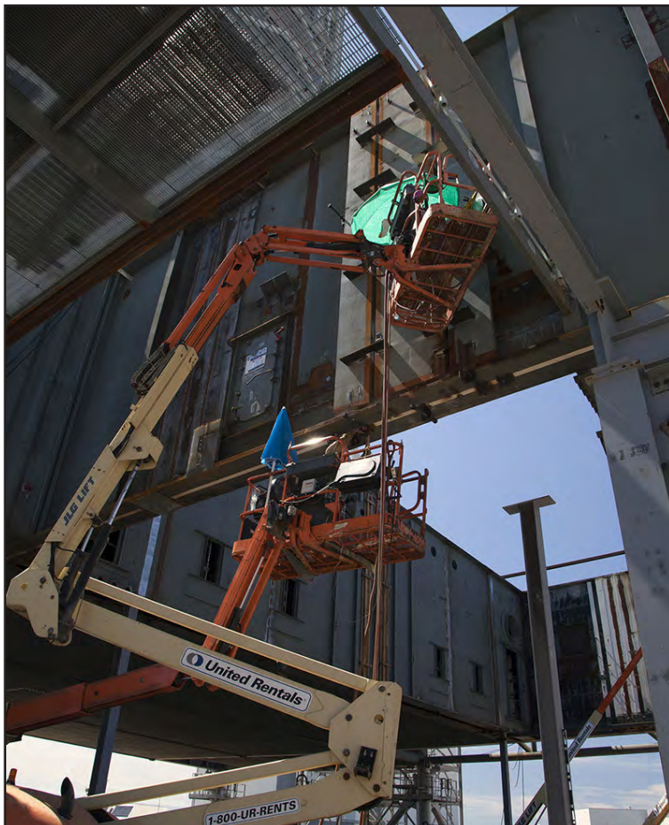
Modifications continued on the Mobile Launcher (ML) on April 22 at the Mobile Launcher Park Site at Kennedy Space Center. Construction workers on lifts prepared to cut and weld sections of the metal walls on the exterior of the ML.
