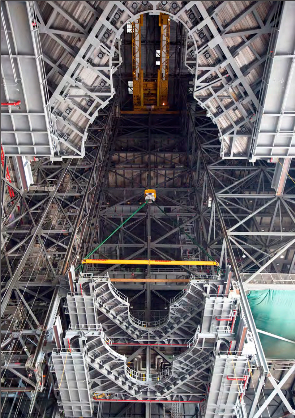
A view from below, in High Bay 3 inside the VAB shows three work platforms installed for NASA's SLS rocket. The lower platforms are the K-level work platforms. Above them are the J-level work platforms. A crane is lowering the second half of the J-level platforms for installation about 112 feet above the floor, or nearly 11 stories high. Photo credit: NASA/Dimitri Gerondidakis
