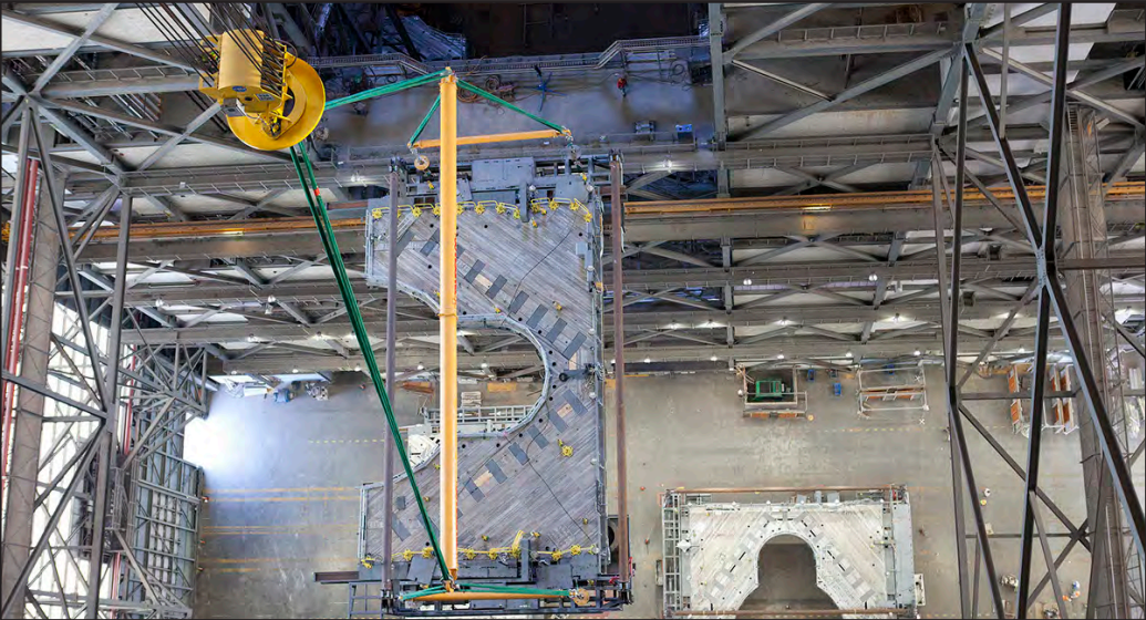
A view from high above inside the VAB shows the first half of the J-level work platforms for the agency's SLS rocket lifted by crane April 5 for installation in High Bay 3. Photo credit: NASA/Glenn Benson
