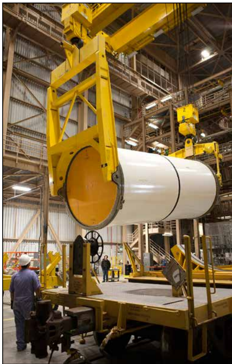
Inside the Rotation, Processing and Surge Facility high bay at NASA's Kennedy Space Center in Florida, engineers and technicians with Jacobs Engineering on the Test and Operations Support Contract monitor the progress Feb. 25 as two cranes are used in tandem to lift the first of two pathfinders, or test versions, of solid rocket booster segments for NASA's SLS rocket. Photo credit: NASA/Ben Smegelsky
