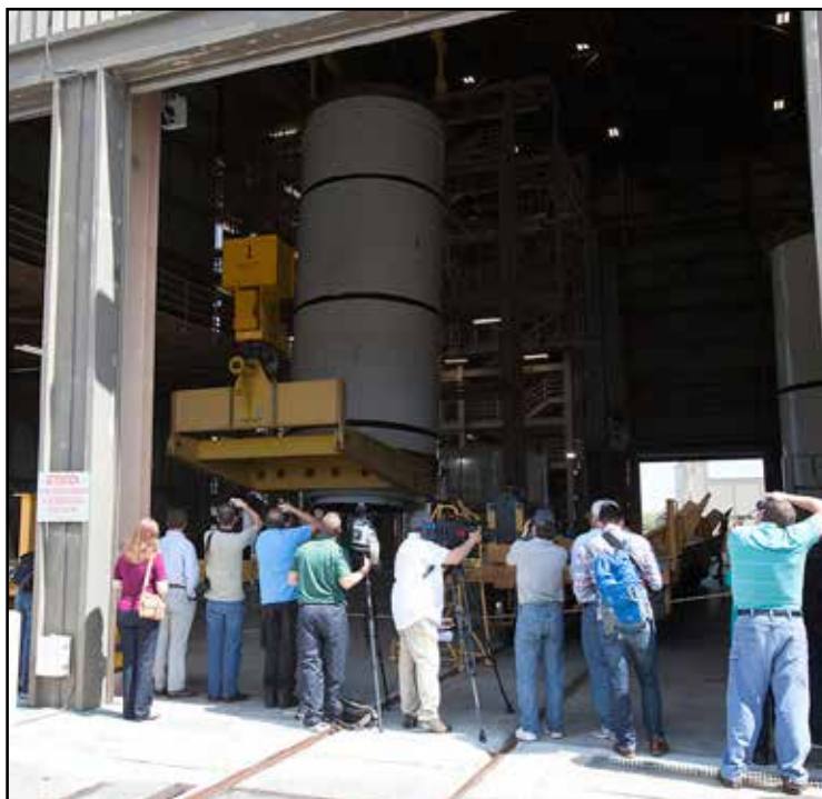
Members of the news media watch March 1 as two cranes are used to lift one of two pathfinders, or test versions, of solid rocket booster segments for NASA's SLS rocket into the vertical position inside the Rotation, Processing and Surge Facility at NASA's Kennedy Space Center in Florida. Photo credit: NASA/Bill White
