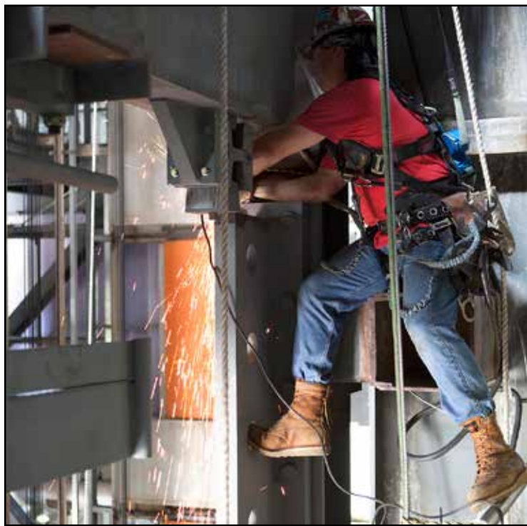
A construction worker, wearing safety gear and tethered to safety lines, works on one of the bolts during installation of the second half of the J-level work platforms April 15. Photo credit: NASA/Dimitri Gerondidakis
