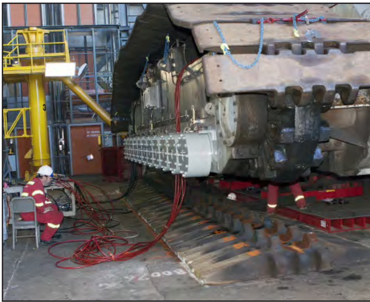
Inside the Vehicle Assembly Building at Kennedy Space Center, preparations are underway to lower crawler-transporter 2 from jack stands so that work can begin to reinstall the large crawler tracks on Dec. 3. The crawler is being prepared for rollout in January 2014 to test the new bearings that were recently installed.
