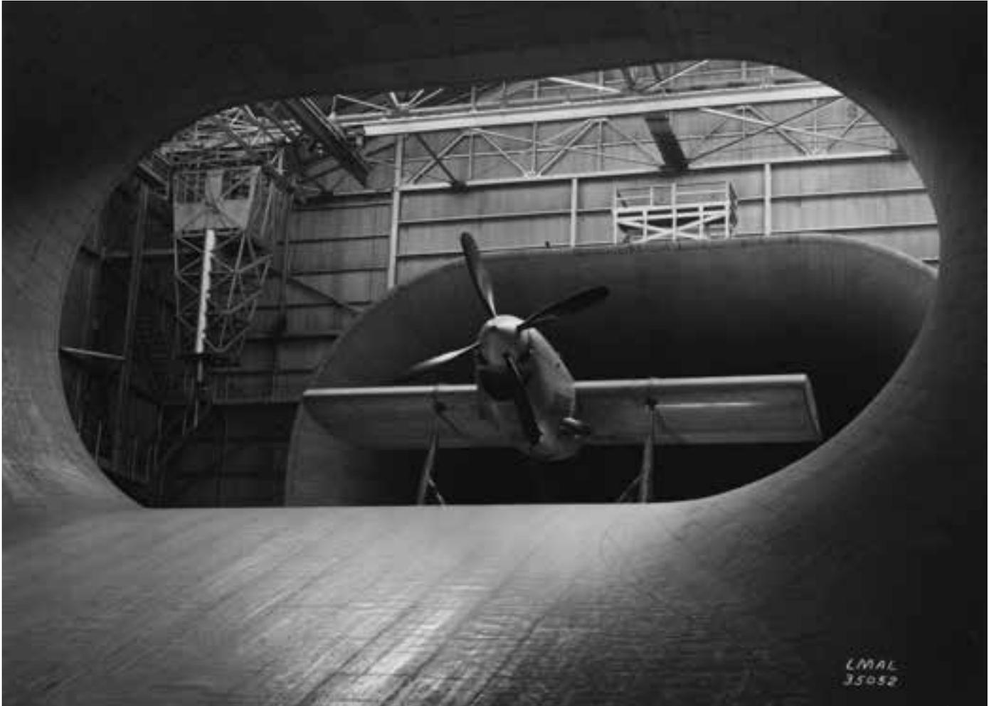
Tests of the Boeing XB-39 engine and engine-nacelle components were conducted in the Full-Scale Tunnel (upper photo) in October 1943 as well as at an outdoor ground facility (bottom photo) in 1944. The test setup and procedure was very similar to those used in B-24D engine tests of 1942. Note the data-acquisition and engine-control rooms at the outdoor site. (NACA LMAL 35052 and NACA LMAL 37951)
