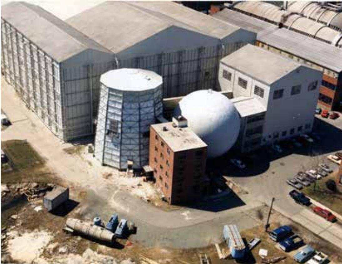
The Langley 12-Foot Free-Flight Tunnel was located in a sphere adjacent to the Full-Scale Tunnel building. In this 1985 aerial photo, facilities include (from top clockwise) the Full-Scale Tunnel, the building that housed the original 15-Foot Free-Spinning Tunnel, the 12-Foot Free-Flight Tunnel, and the 20-Foot Spin Tunnel. The Langley 16-Foot Transonic Dynamics Tunnel (TDT) is at the extreme upper right. (NASA L-85-3591)
