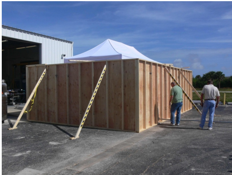
Test Unit Plywood Protective Barrier Under Construction
