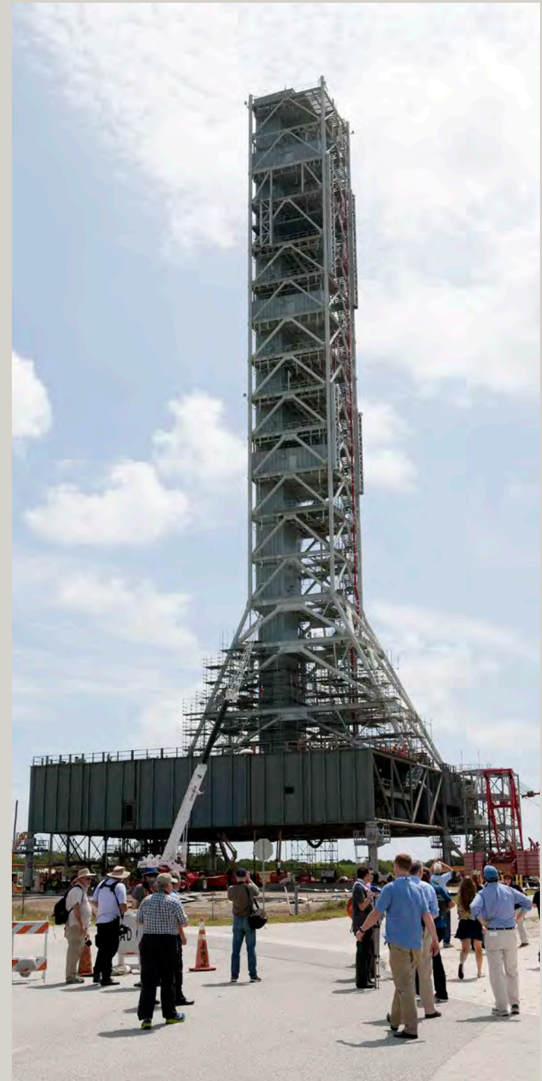
The mobile launcher, or ML, that will support NASA's Space Launch System, or SLS, and Orion spacecraft for Exploration Mission-1 is in view at the Mobile Launcher Park Site at Kennedy Space Center. The ML base and tower structure were modified to accommodate the weight, size and thrust at launch of the SLS and Orion spacecraft. Photo credit: NASA/Cory Huston
