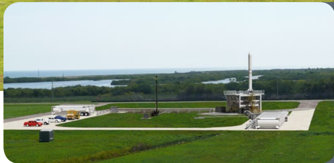
A new Small Class Vehicle Launch Pad, designated 39C, is being constructed in the southeast area of the perimeter of Launch Pad 39B at Kennedy Space Center. This computer-aided view shows the new concrete pad, universal propellant servicing system, and customer-provided launch mount. Image credit: David Zeiters
