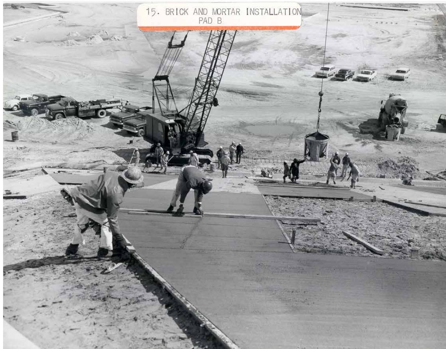
Pouring concrete at Launch Pad 39B on March 7, 1966. Photo credit: NASA
