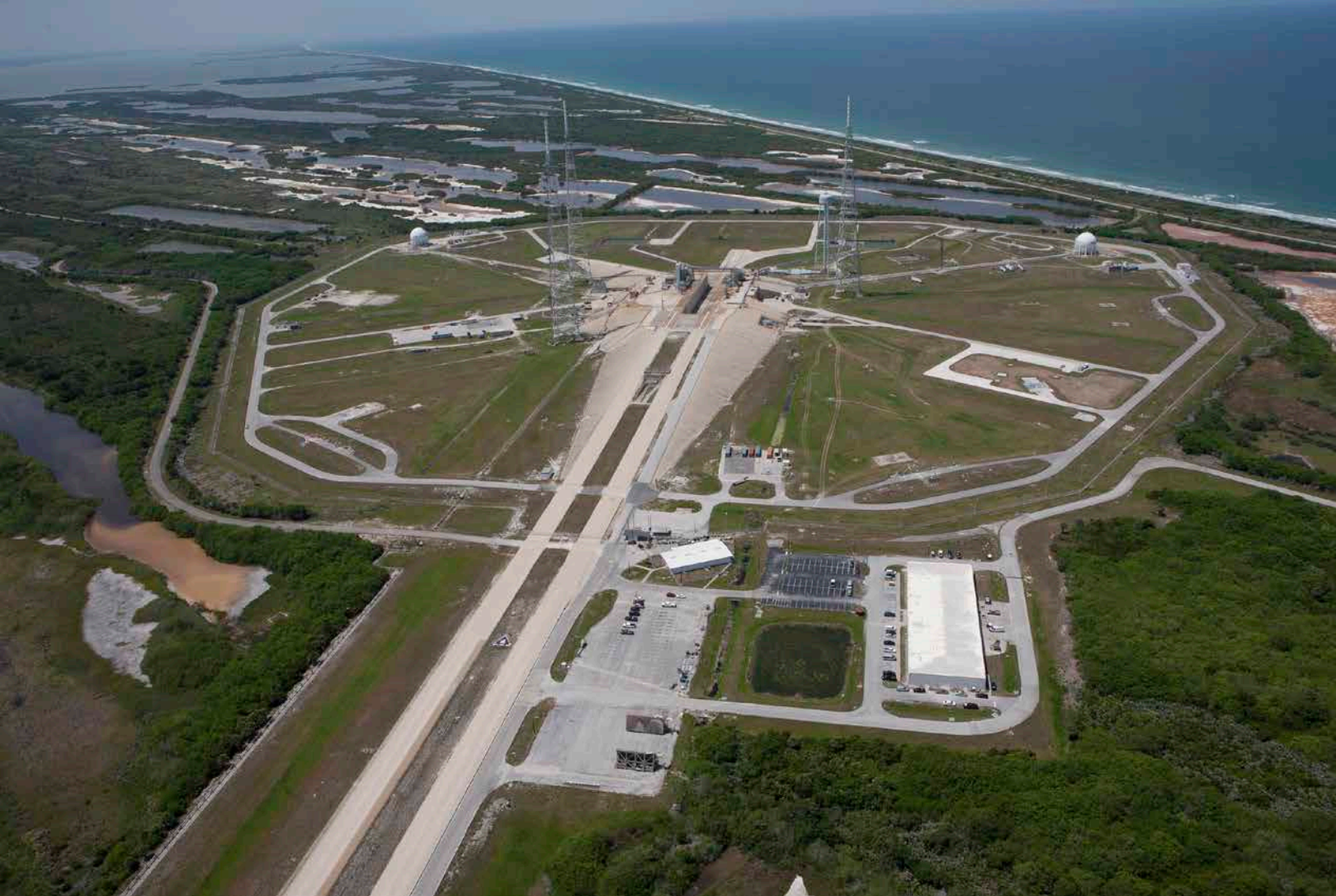
An aerial view of Launch Complex 39B at Kennedy Space Center. Photo credit: NASA/Kim Shiflett
