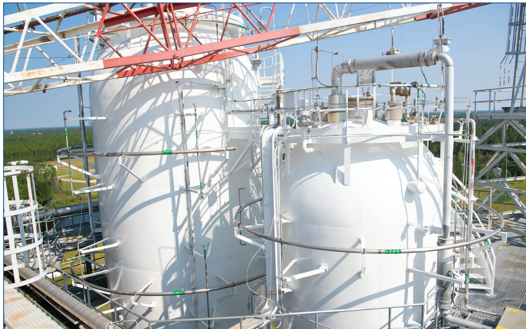
A recent photo shows the recoated and newly serviced liquid hydrogen and liquid oxygen run tanks on the A-1 Test Stand at Stennis. The project was one of several to prepare the historic Stennis stand for a new series of RS-25 engine tests.
