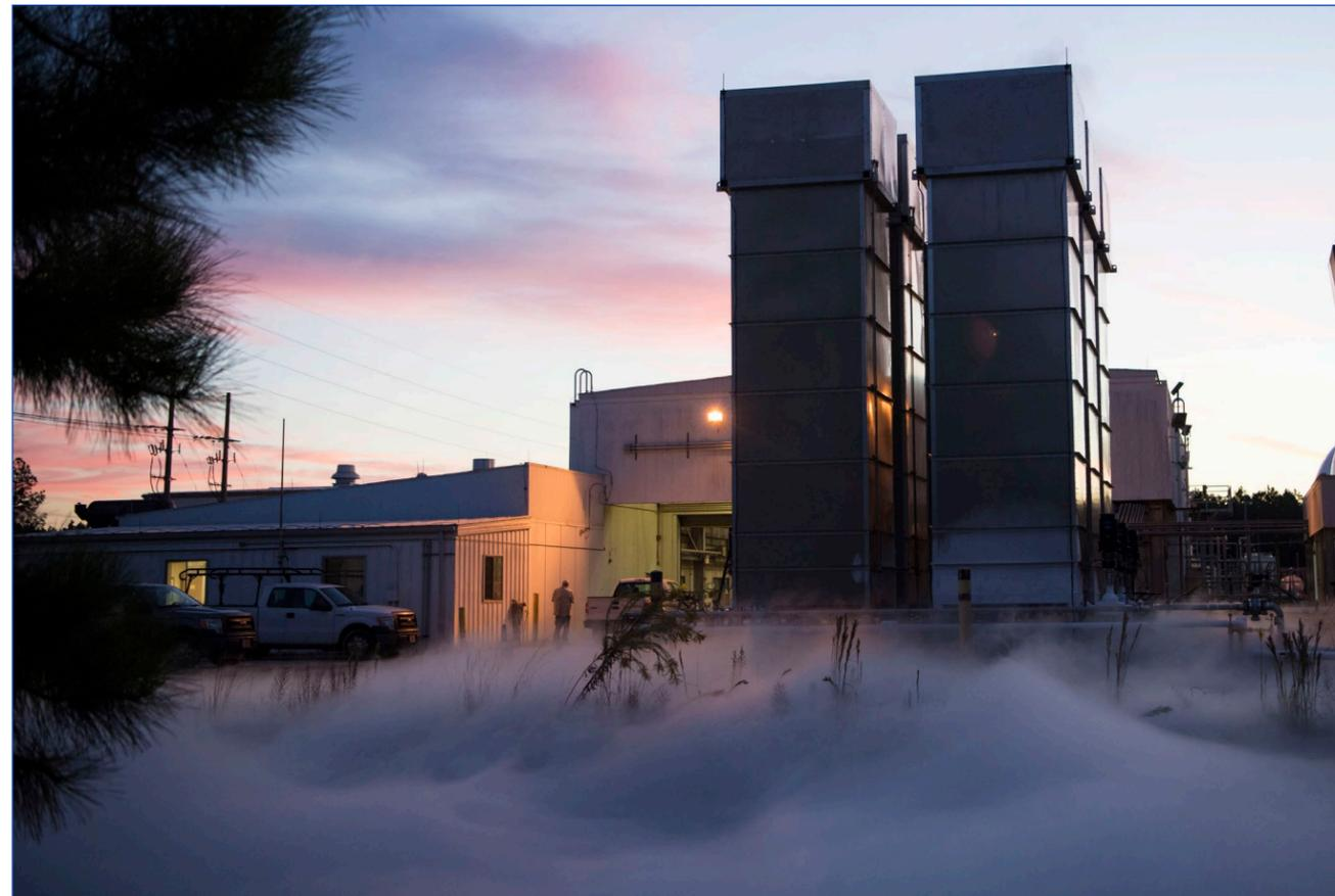
The Stennis high-pressure gas facility produces four high-pressure gases for testing and maintaining test systems. Compressors pump low-pressure helium and atmospheric air up to high-pressure levels. Vaporizers convert liquid nitrogen and liquid hydrogen to high-pressure gases. All four are needed for SLS testing.
