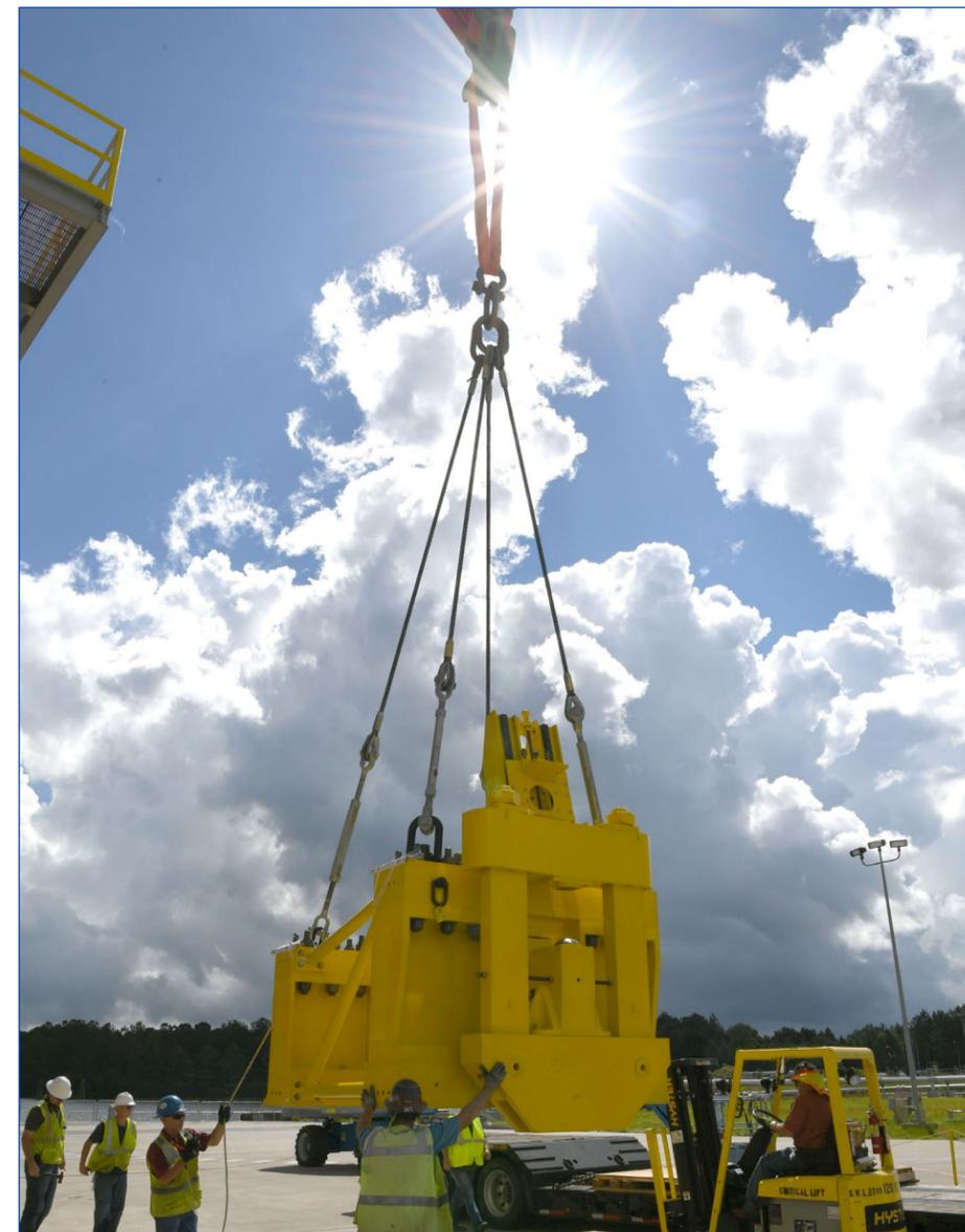
B-2 Test Stand team members prepare to lift one of two so-called "yellow boxes" onto the stand for installation. The yellow boxes will help anchor NASA's Space Launch System core stage in place during testing.
